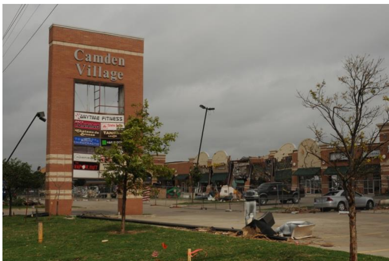
Figure 2: Shopping Mall Damaged by a Tornado (FEMA Photo by George Armstrong)
