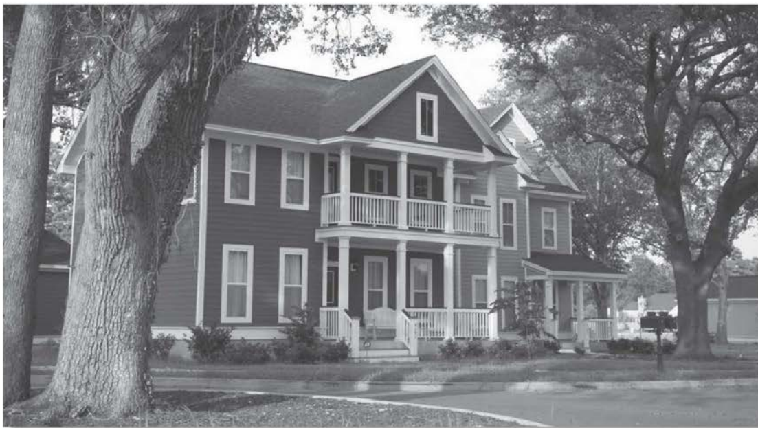
The Oak Terrace Preserve community in North Charleston, S.C., was zoned and permitted under a PUD ordinance that allowed the developers to employ LID principles in the development and preserve up to 95% of the older, healthy trees on site. Photo/City of North Charleston
