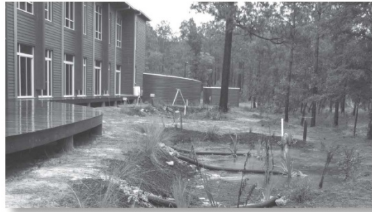
Researchers from Clemson University have recently designed, installed, and are currently studying water retention capacity and performance of bioretention cells at their new Baruch Institute facility in Georgetown, S.C. Photo/Clemson University
