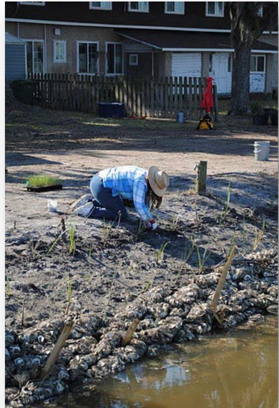
Volunteer installing bagged oyster shells and marsh plantings. Source: Jan Mackinnon
