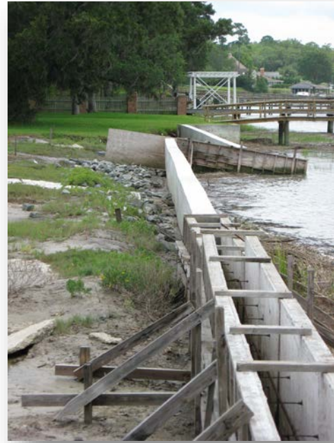
Typical Concrete Bulkhead Construction. Source: Dr. Clark Alexander
