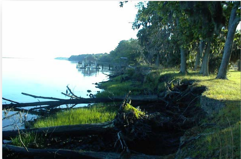
Bank Erosion on St. Catherines Island. Source: Tara Merrill
