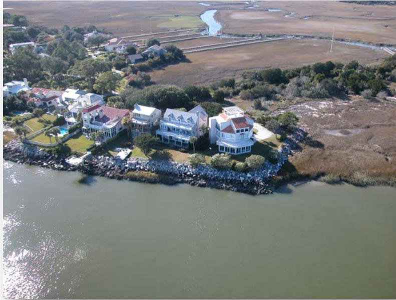
Typical Coastal Development with Structural Stabilization Measures (Bulkheads/Rip Rap Revetment). Source: Dr. Clark Alexander
