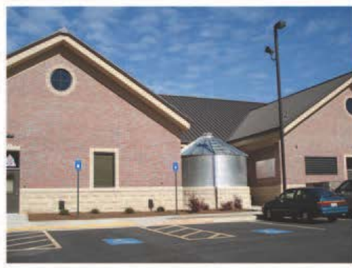
The Emergency Operations Center in Douglas County collects and stores rainwater.
