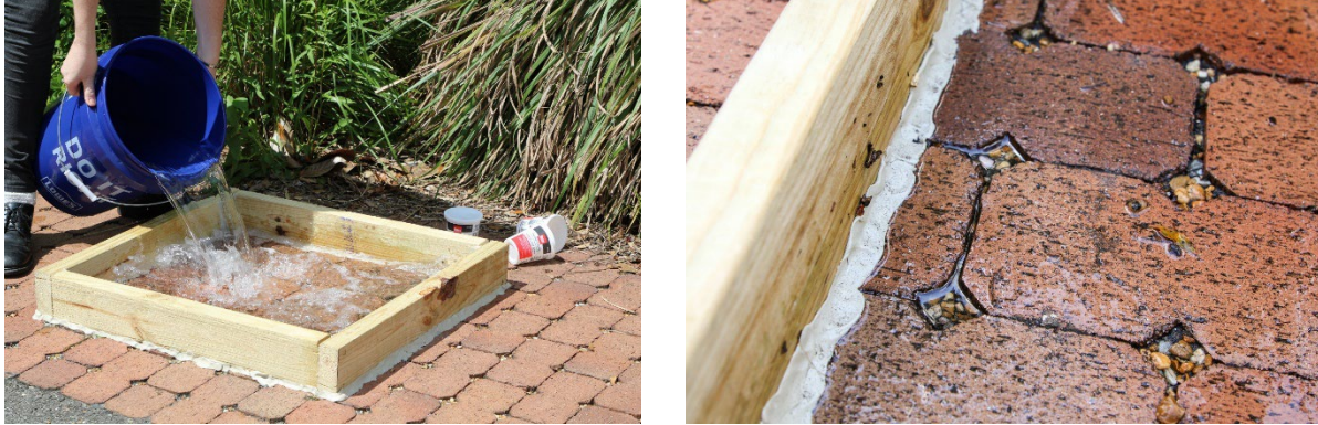
Figure 3. SIT Testing (water added on left, end of test on right)
