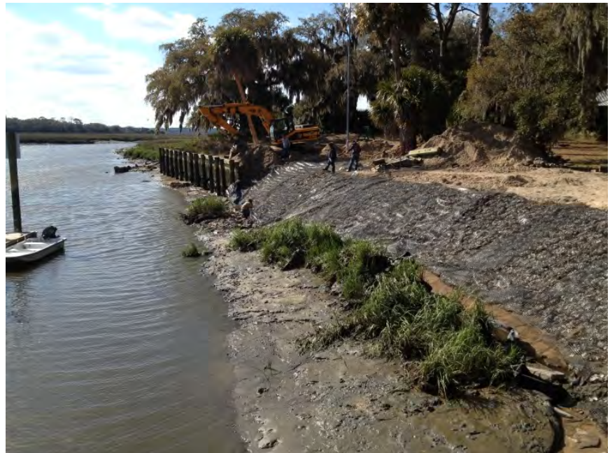
Bottom course of oyster bags wrapped in geogrid after bulkhead removal. Little St. Simons Island, GA.
