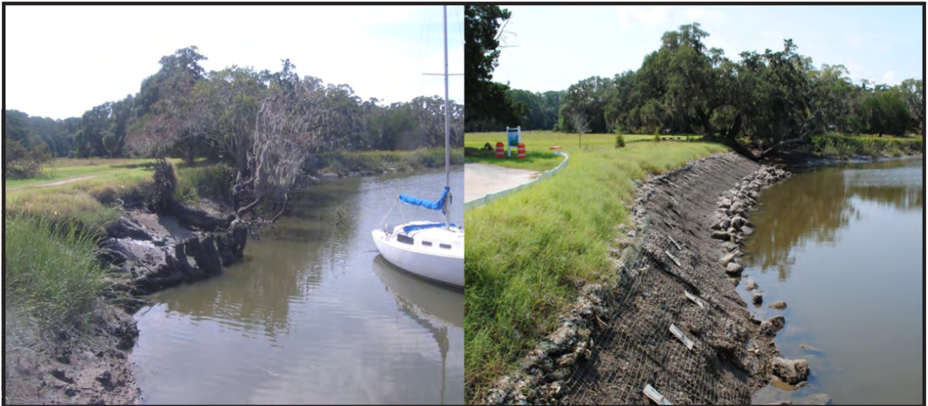
Long Tabby Living Shoreline pre-construction in 2009 (left) and post-construction in 2010 (right)
