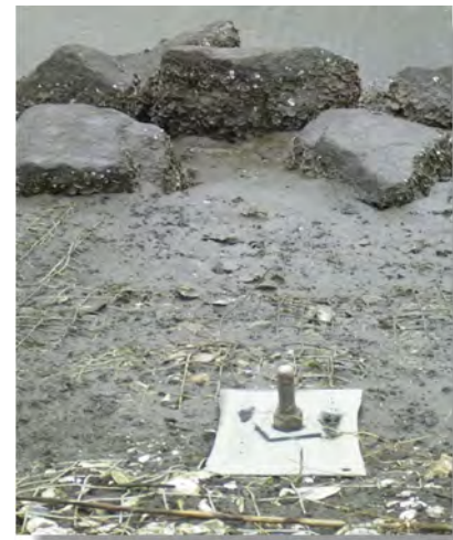
Figure 2. Gabion with anchor and rock toe.
