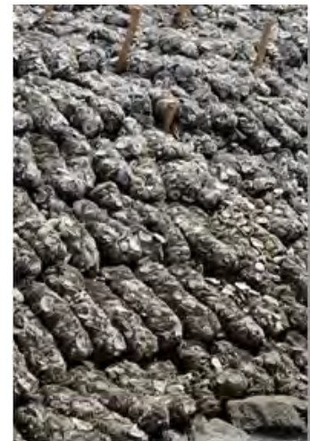
Detail of Ashantilly site oyster bag placement
