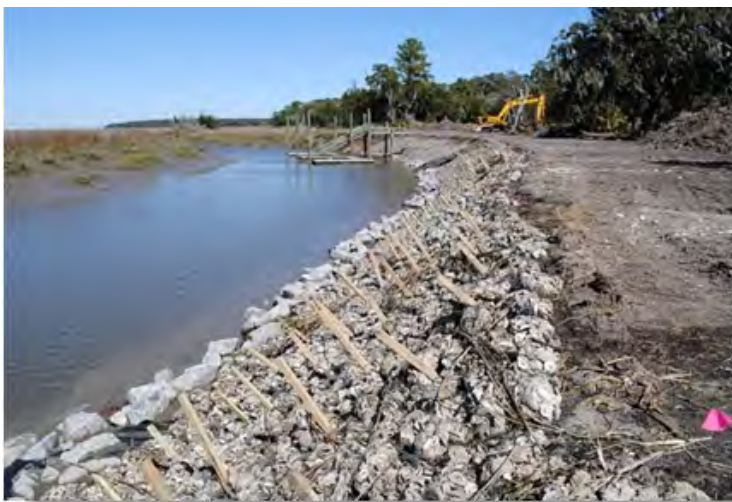
Ashantilly site construction photo
