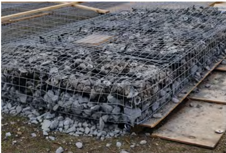
Figure 1. Gabion basket filled with granite and a bagged shell laminate.
