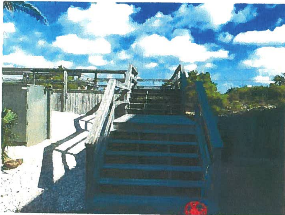
Figure 1 - Steps leading to boardwalk. 6.5' wide with 6" outside handrails.
