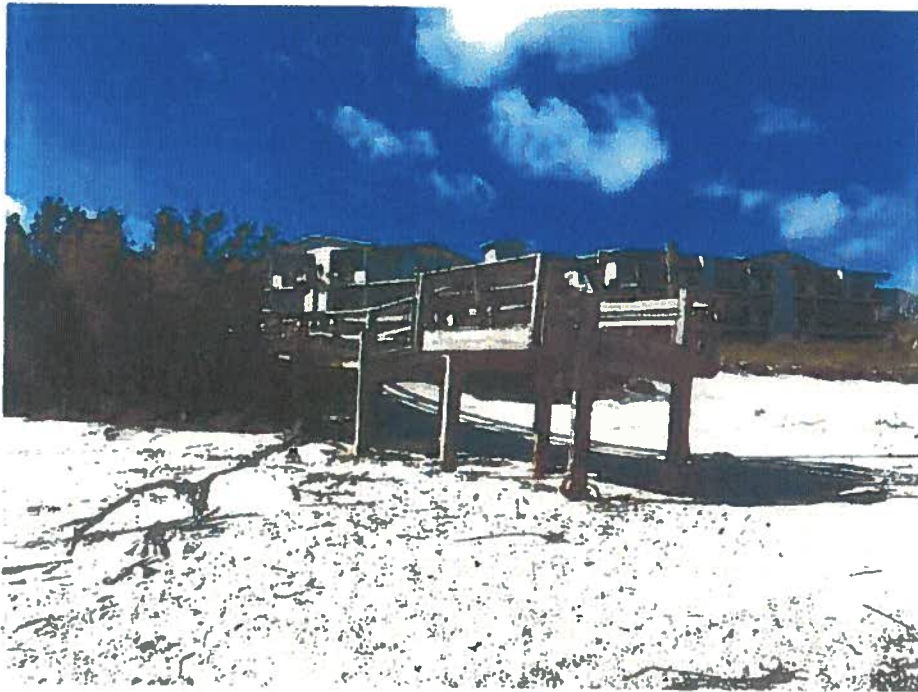
Figure 6 - Beach view of damaged boardwalk and deck
