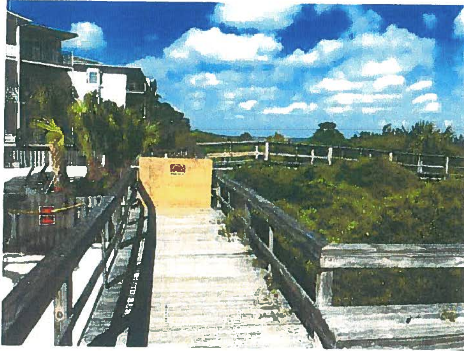
Figure 3 - Looking west along boardwalk parallel to beach. 6.5' walk with 6" outside handrails.
