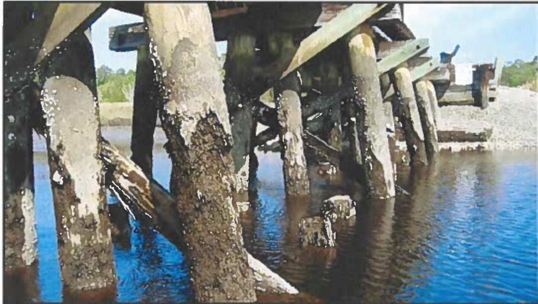
Figure 4 Detail of Pilings, View Looking Northeast.
