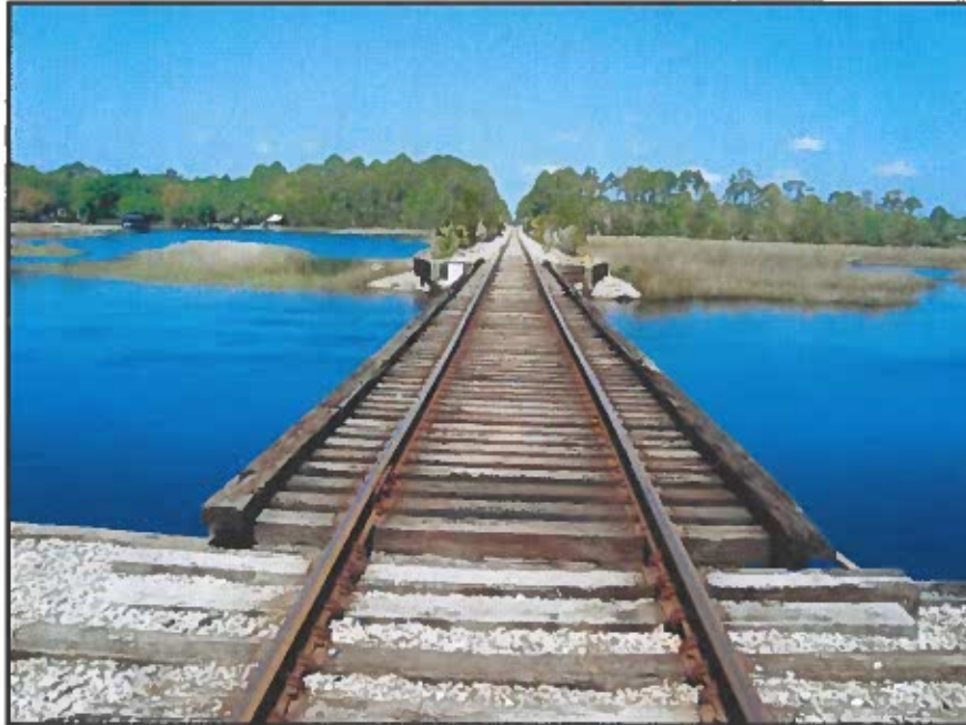
Figure 2 Overview of Bridge, Looking Northwest.
