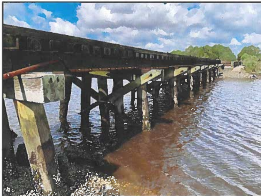
Figure 3 Overview of Bridge, Looking West.
