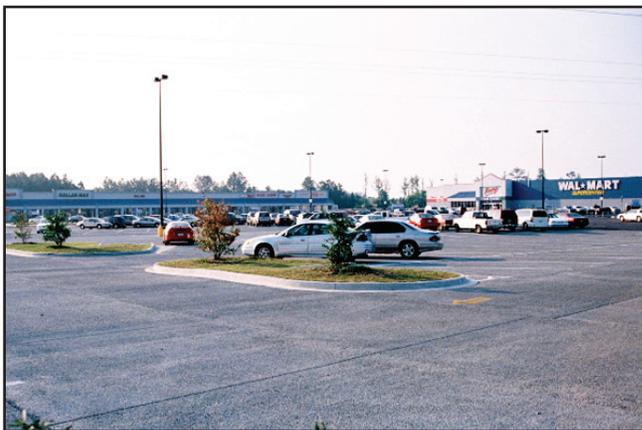
*Figure 3.3.8a Pervious Concrete Used in Wal-mart Parking Lot*
