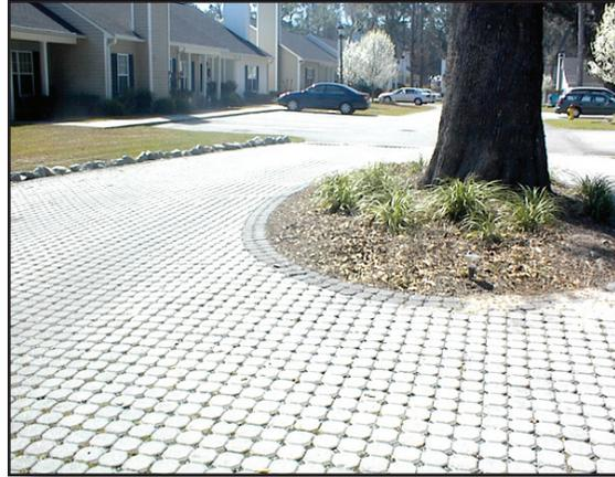
*Figure 3.3.8d Permeable Pavers Around Parking and Drive Areas*
