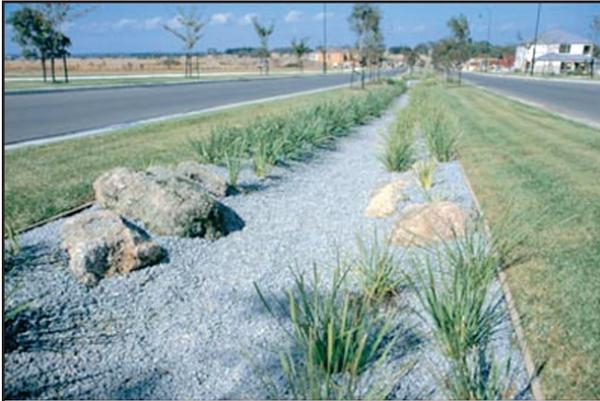
*Figure 3.3.5a Infiltration Trench in Highway Median*
