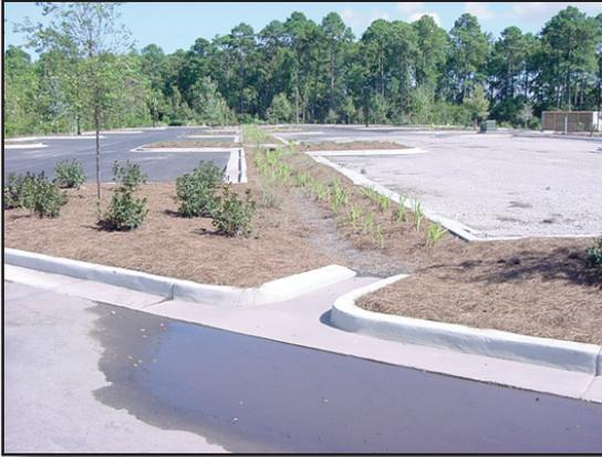
Figure 3.3.4b Bioretention Swales with Curb Cut
