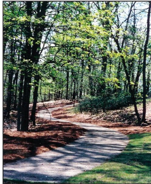
*Figure 3.3.8e Pervious Concrete Pathway Dyed to Match Native Soils*
