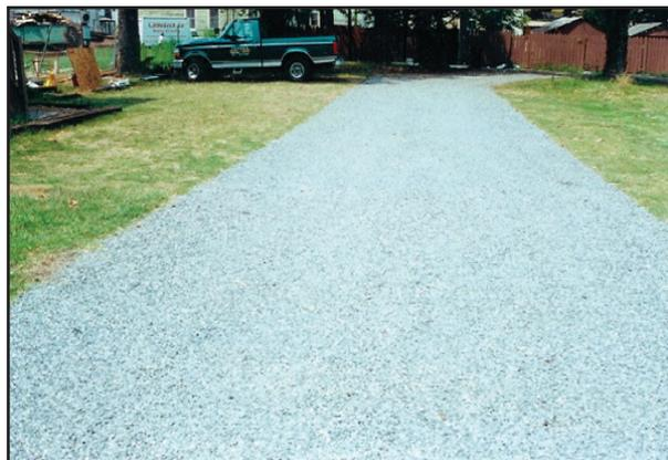
*Figure 3.3.8f Gravel Pave and Slope Tame on Residential Diveway*
