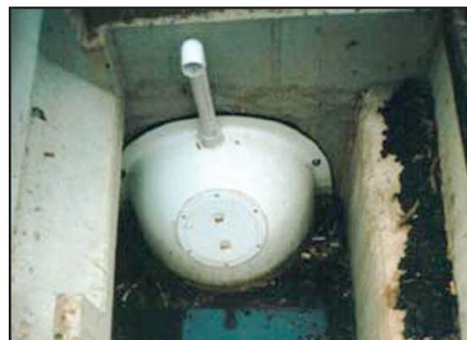
Figure 3.3.9d Snout Structure in Place
