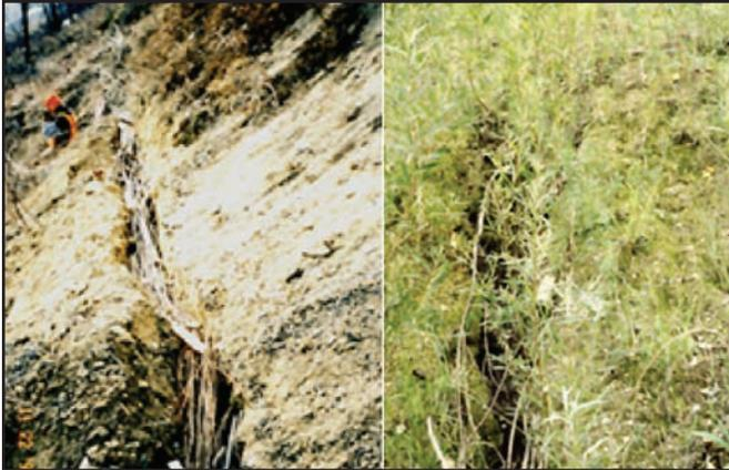
*Figure 4.5.8a Brush Trench with Willow Cuttings During and After Construction*
