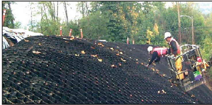
*Figure 4.5.11d Installation of GeoWeb*
