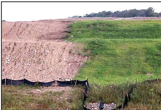
*Figure 4.2.1a Vegetated Slope vs. Non-vegetated Slope with Rills and Gullies*
