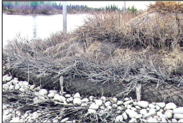
Figure 4.5.6a Initial Installation of Brush Layering
