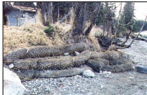
*Figure 4.5.3d Installation of Straw and Coir Log Along Stream Bank at Low Tide
