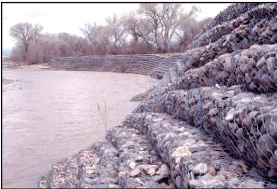
*Figure 4.5.9a Tiered Installation of Rock Gabions*
