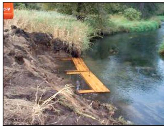
*Figure 4.5.11f Fish Lunker Structure*
