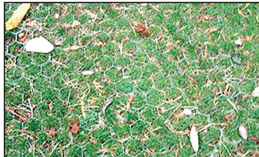
*Figure 4.5.4c Hexagonal Cells Filled with Turf for Bank Reinforcement*
