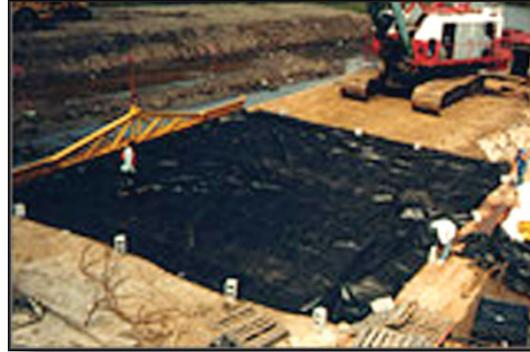
*Figure 4.5.4a Filter Fabric Applied to a Moderate Slope*
