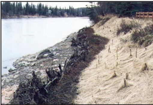
*Figure 4.5.3a Coconut Mat on Stream Bank
