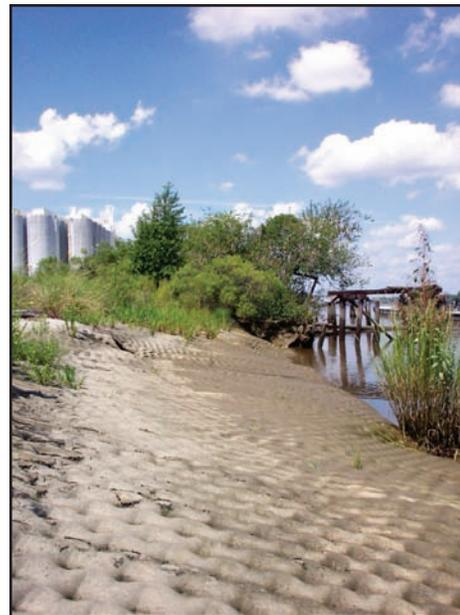
*Figure 4.5a Hard Armoring of Bank Which Prohibits Native Vegetation, Degrades Wildlife Habitat, and Deters Infiltration of Stormwater
