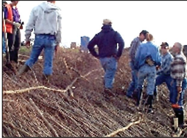
*Figure 4.5.7a Brush Mattresses Being Installed*
