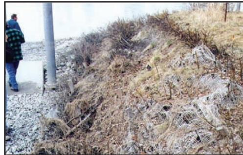
*Figure 4.5.3b Biodegrading Coconut Mat Along Bank
