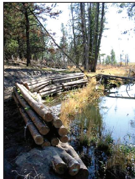
Figure 4.5.11b Stream Channel After Log Revetment
