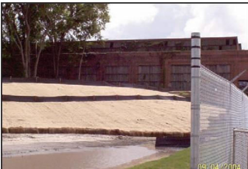
*Figure 4.5.3c Jute Mesh Covering Slope
