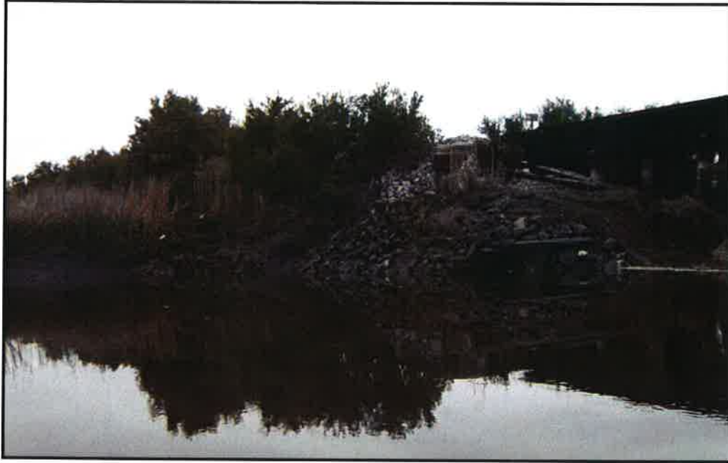
Photo 9– Facing South East End Bent Zero– NE Abutment.
