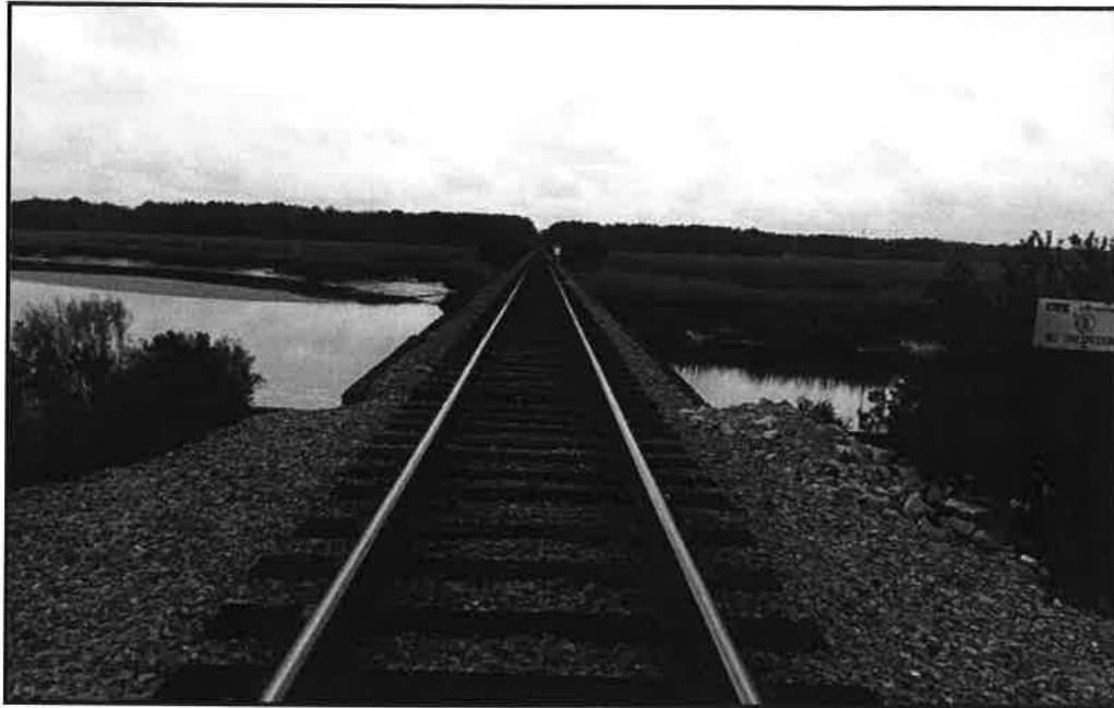
Photo 3– Facing West Along Tracks From East Abutment.
