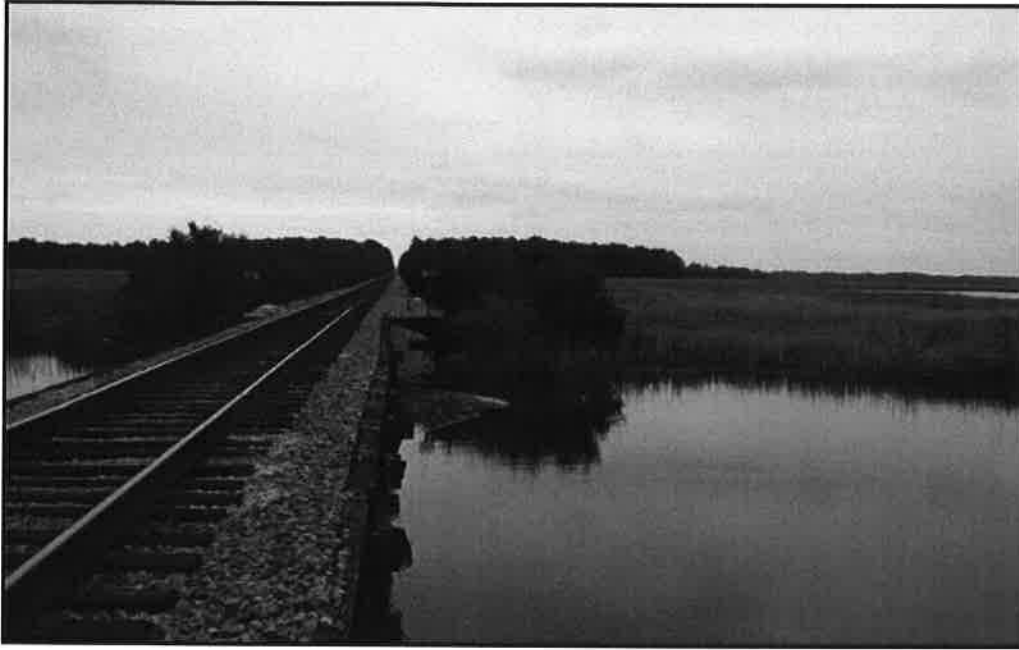
Photo 7— Facing East Along Tracks—Downstream Face.
