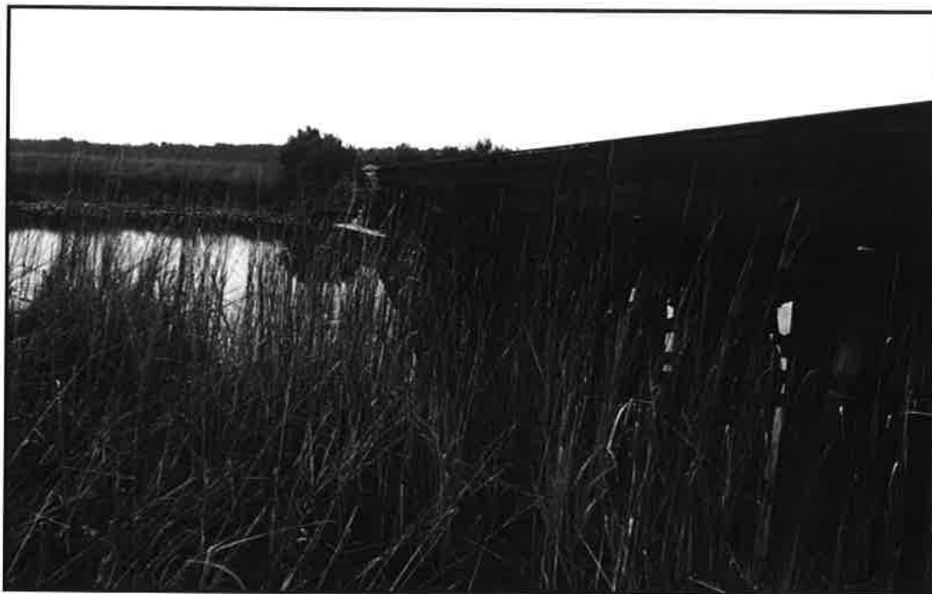
Photo 2– Facing East Along Upstream Face.
