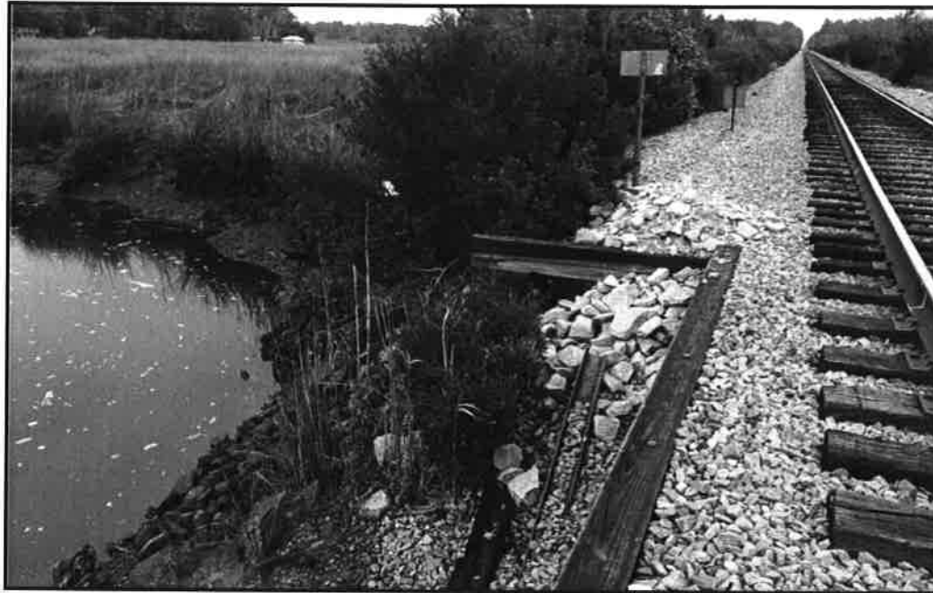
Photo 5- Facing East End Bent Zero- NE Abutment.
