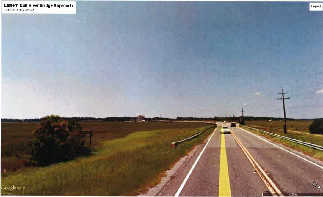
Photograph 2: Eastern end of Bull River Bridge. The approach road for the new bridge will be constructed on southeastern side of the existing road (left side in photograph).
