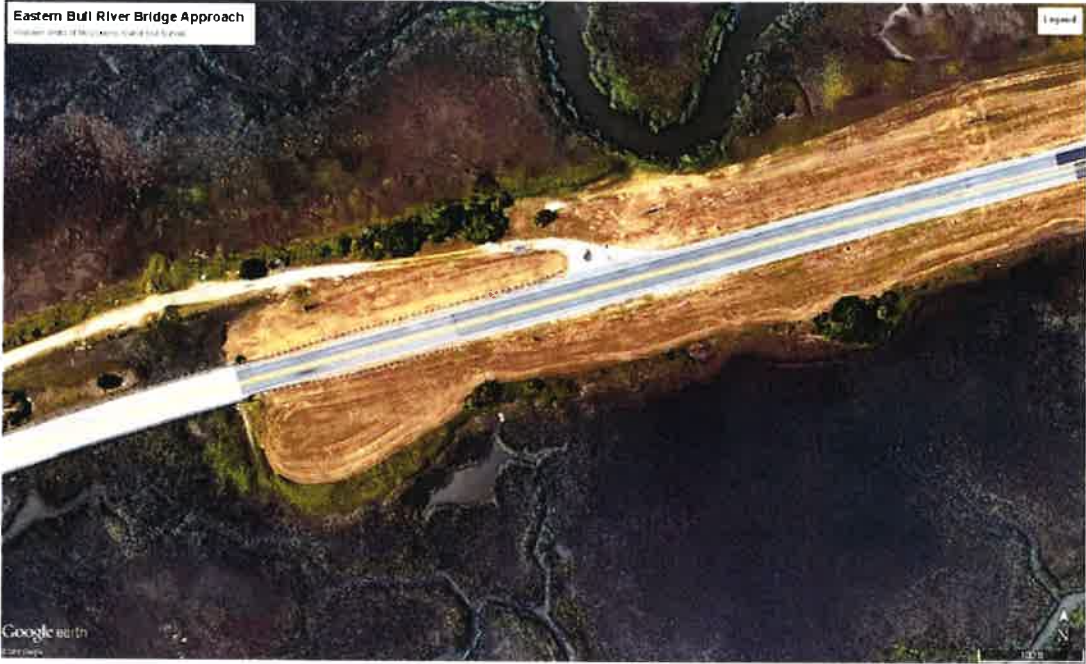
Photograph 1: Eastern end of Bull River Bridge. The approach road for the new bridge will be constructed on southeastern side of the existing road. See Drawings 5 and 6 for boring locations.
