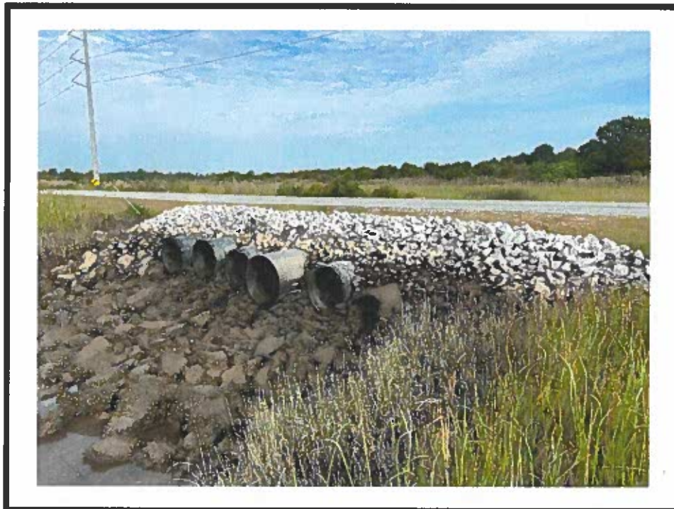
Photo 2: Facing north at Elba Island Rd culverts
