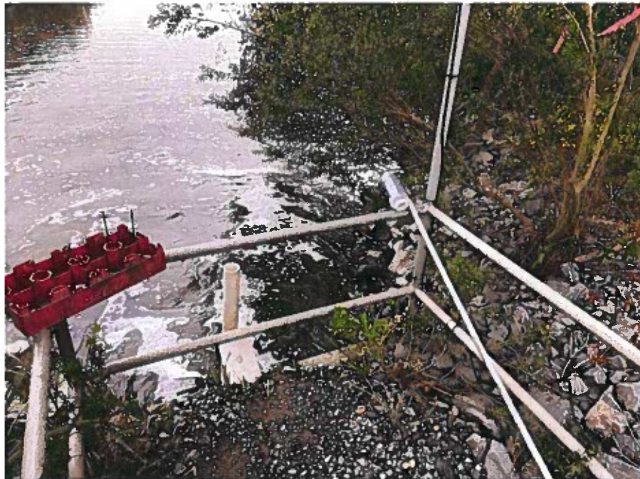
View of existing effluent structure and rip rap-reinforced area facing Southwest.
