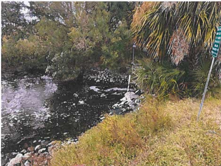
View of existing effluent structure and rip rap-reinforced areas facing West.
