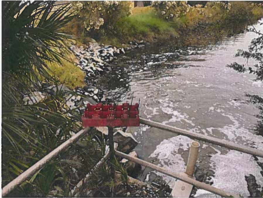
View of existing effluent structure and rip rap-reinforced area facing Southeast.
