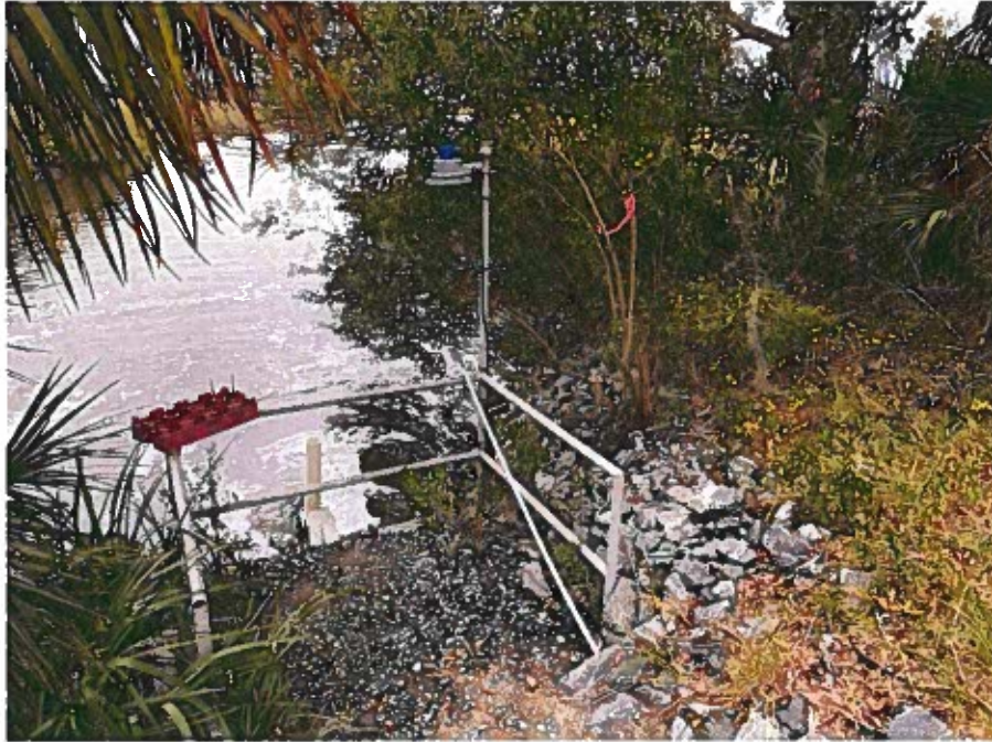
View of existing effluent structure facing Southwest.
