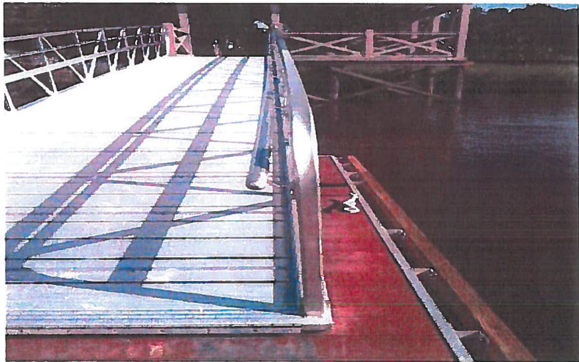
Photograph 2 Gangway With Curb & Railing
