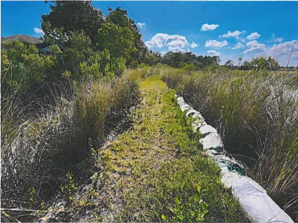
Photo 3: Temporary sandbag barrier installed along dike at location of increased erosion
