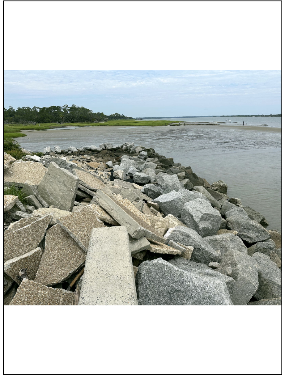
Photo 2: Seaward End of Revetment at Bulkhead (31.214085, -81.311590)
