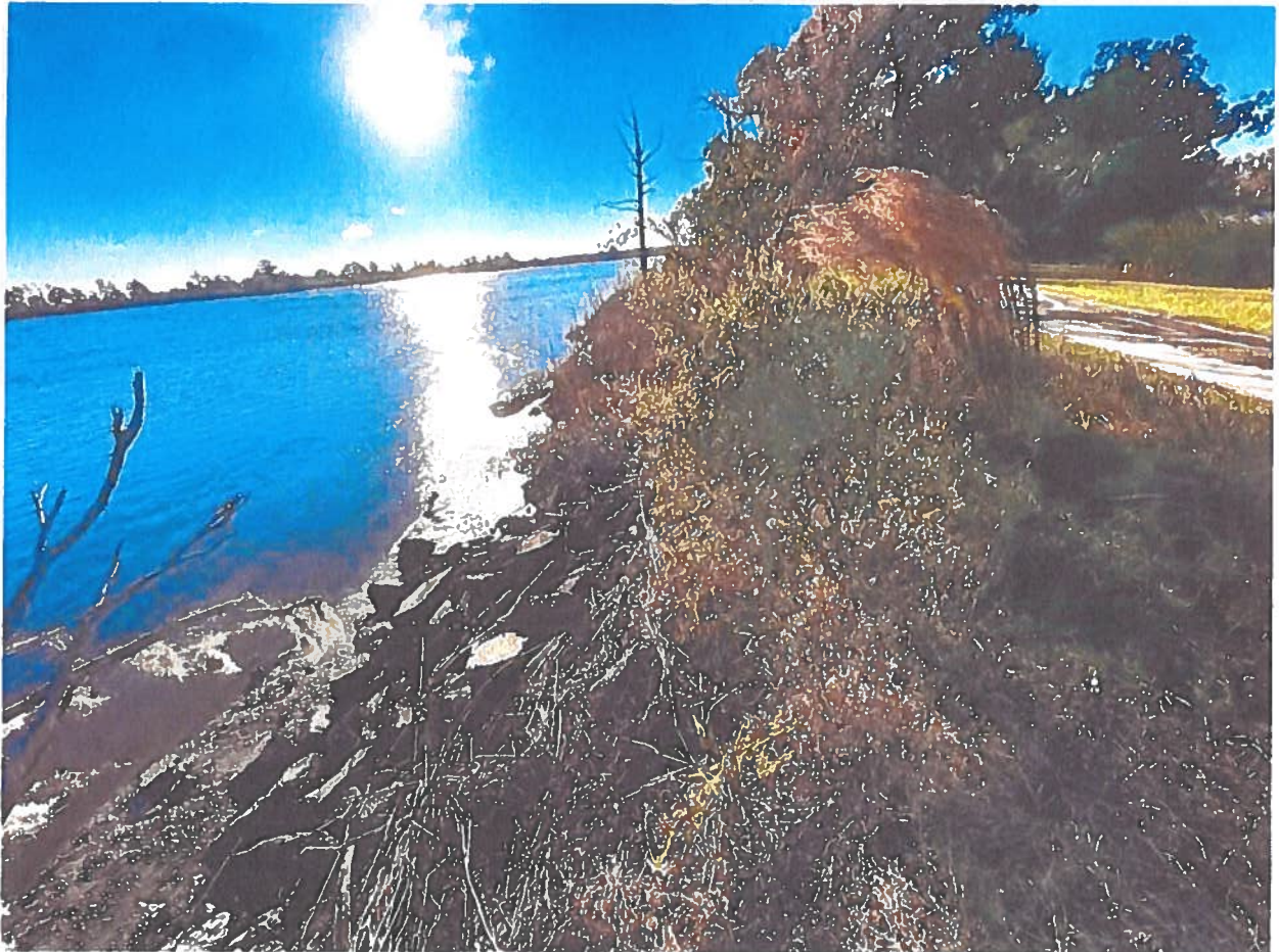
Figure 38. Levee Section Previously Riprapped
