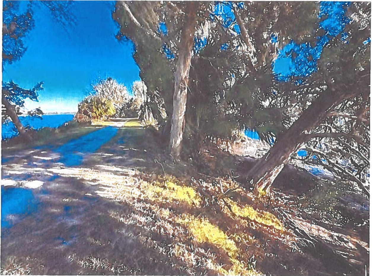
Figure 24. Narrow Section of Levee recommended for riprapping.
