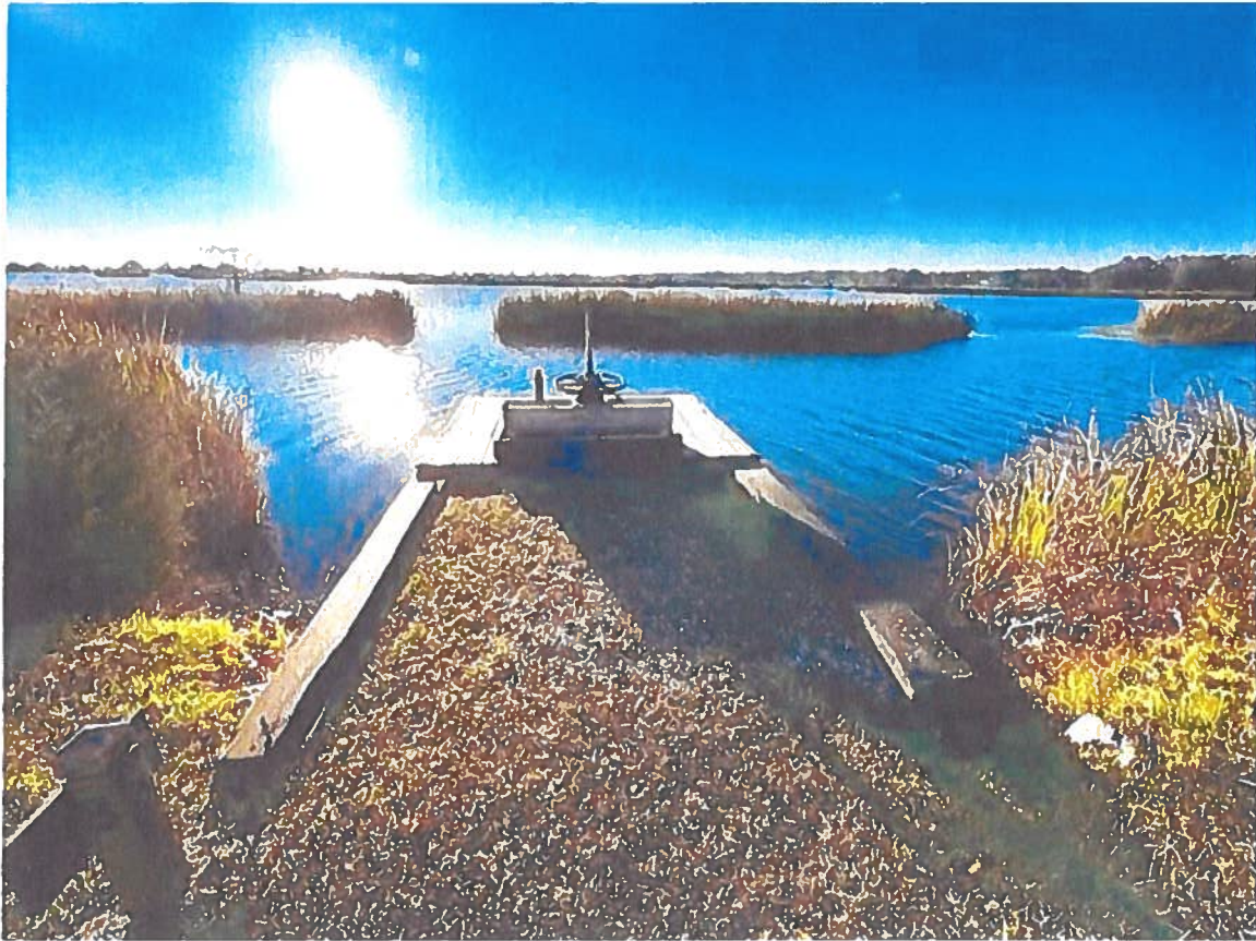
Figure 10. Section of Dike requiring Riprap
