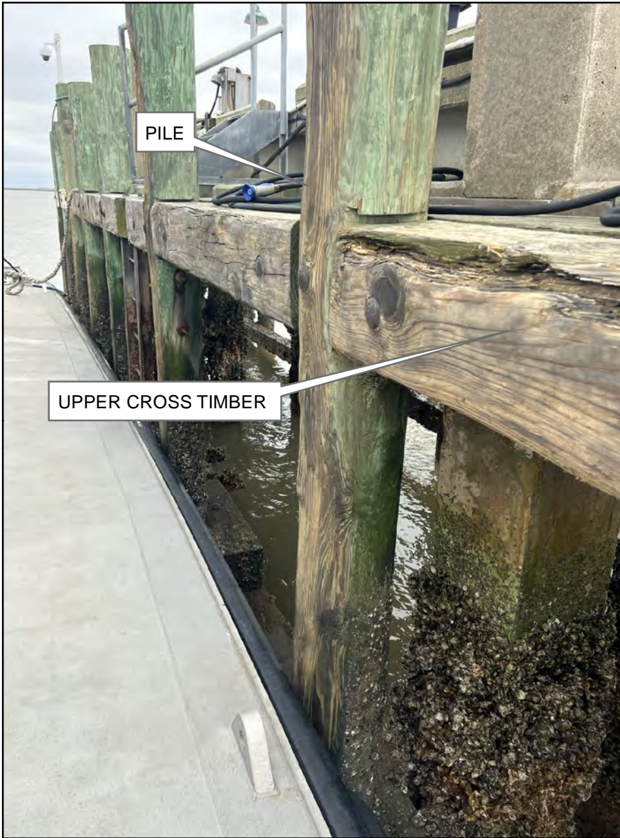
Photo 3: Example of upper cross timber and pile to be replaced
