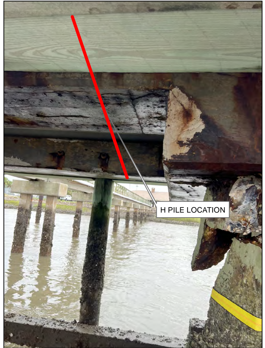
Photo 2: Location for H pile installation next to fractured pile
