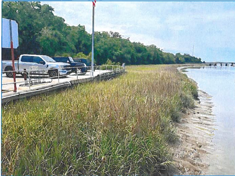
Existing bulkhead and marsh facing south
