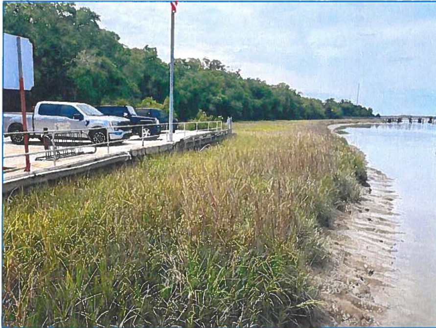
Existing bulkhead and marsh facing south
