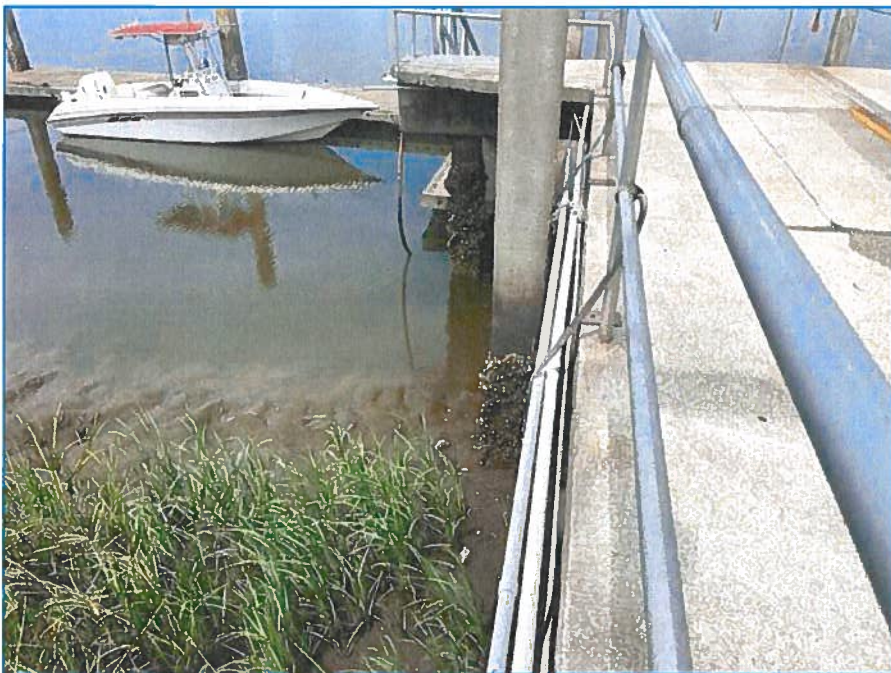
Area for new concrete decking over marsh – 218SF
