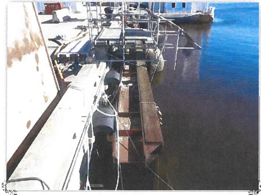
PHOTOGRAPH 1* – View to northeast along the TRF Interface Wharf face (photo left). USACE jurisdiction in this location extends to the Mean High-Water Line (MHWL). The existing brown steel fender system shown water ward of the concrete barrier will be replaced with square concrete piles. No emergent estuarine vegetation or submerged aquatic vegetation occurs waterward of the hardened shoreline within the project area.
