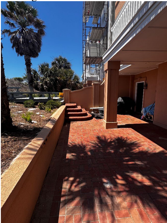
Site Conditions: Ground level
