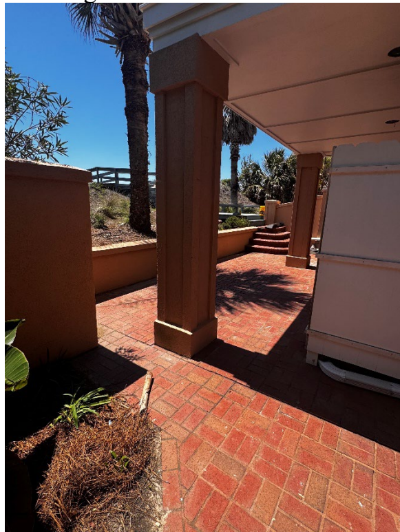
Site Conditions Ground Level
