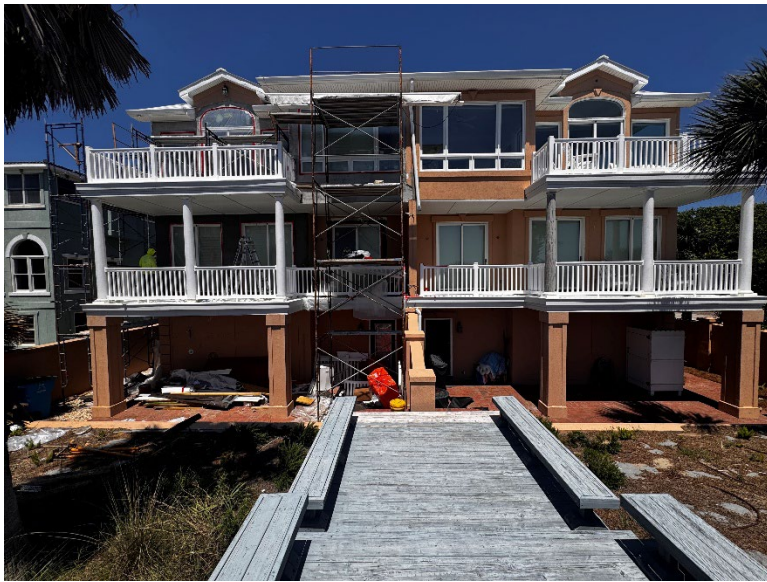
Existing Under Construction Rock Repair
