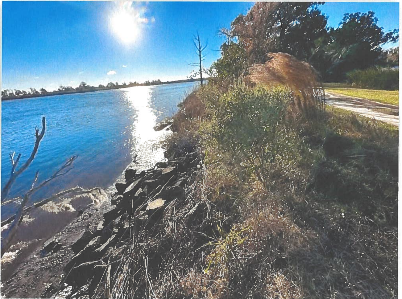
Figure 38. Levee Section Previously Riprapped
