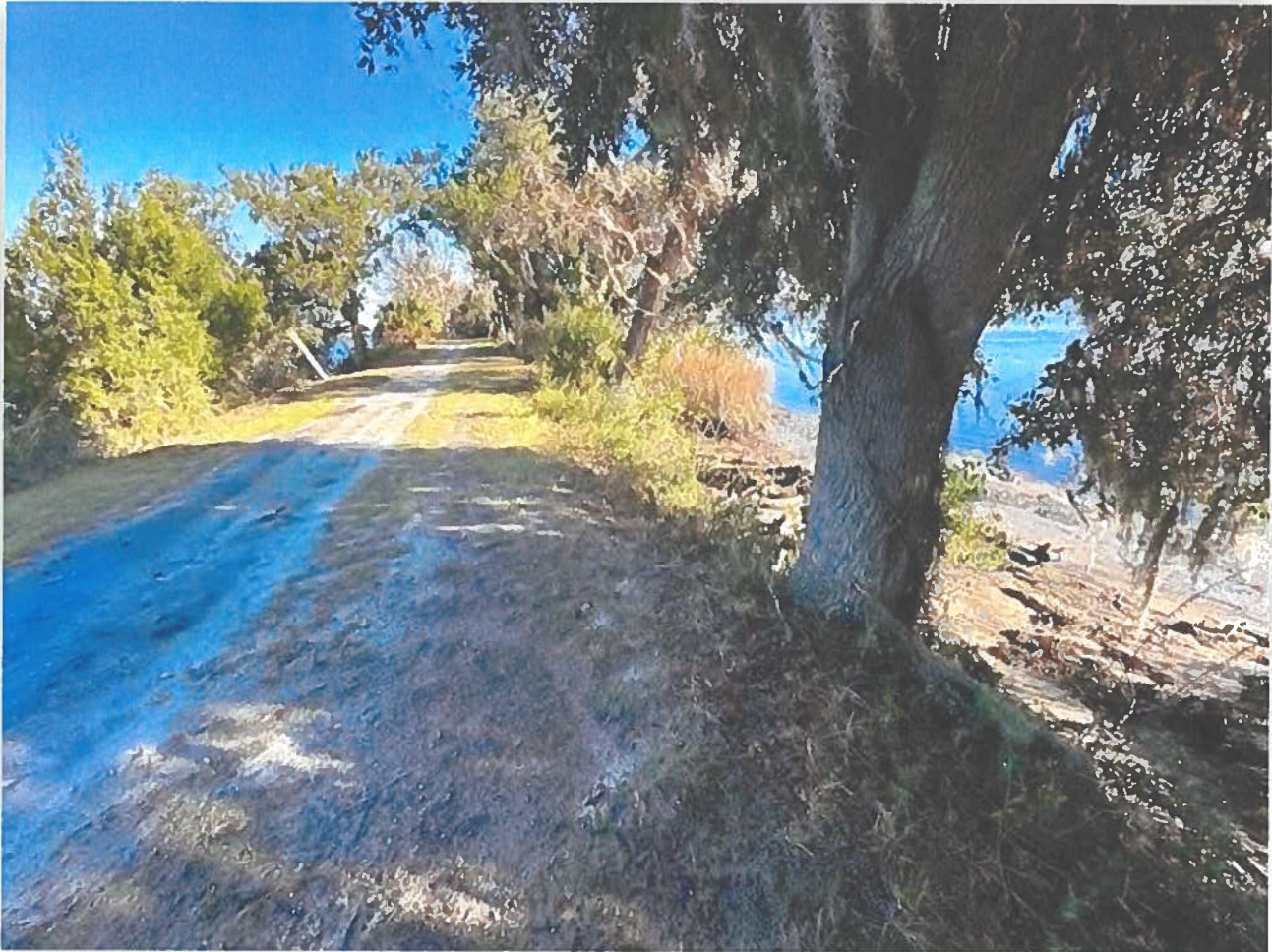
Figure 25. Narrow Section of Levee recommended to be riprapped.
