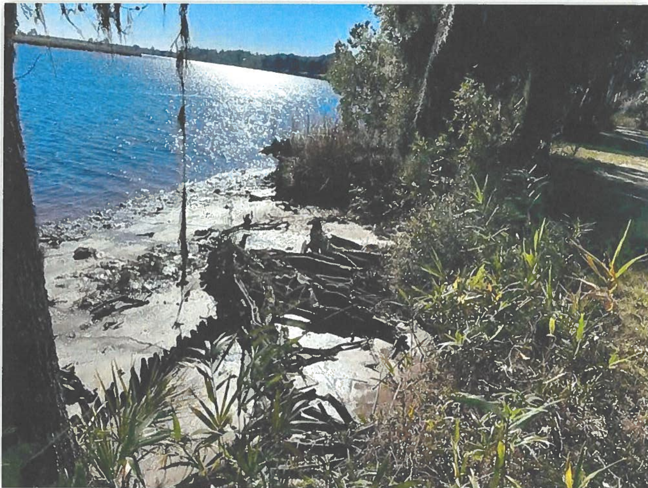
Figure 35. Remnants of Timber Retaining Wall
