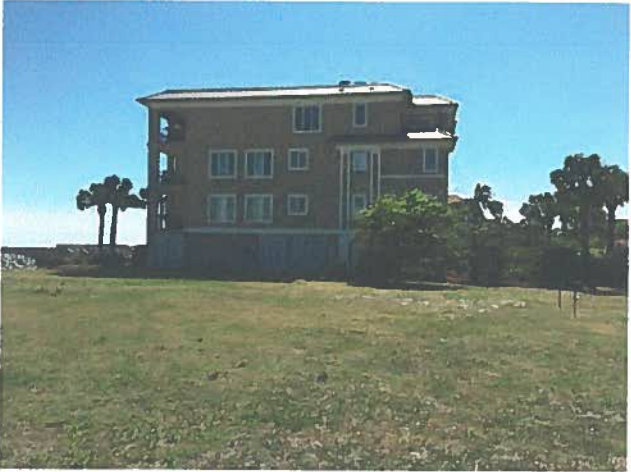
View of site looking towards Marbella Condominium
