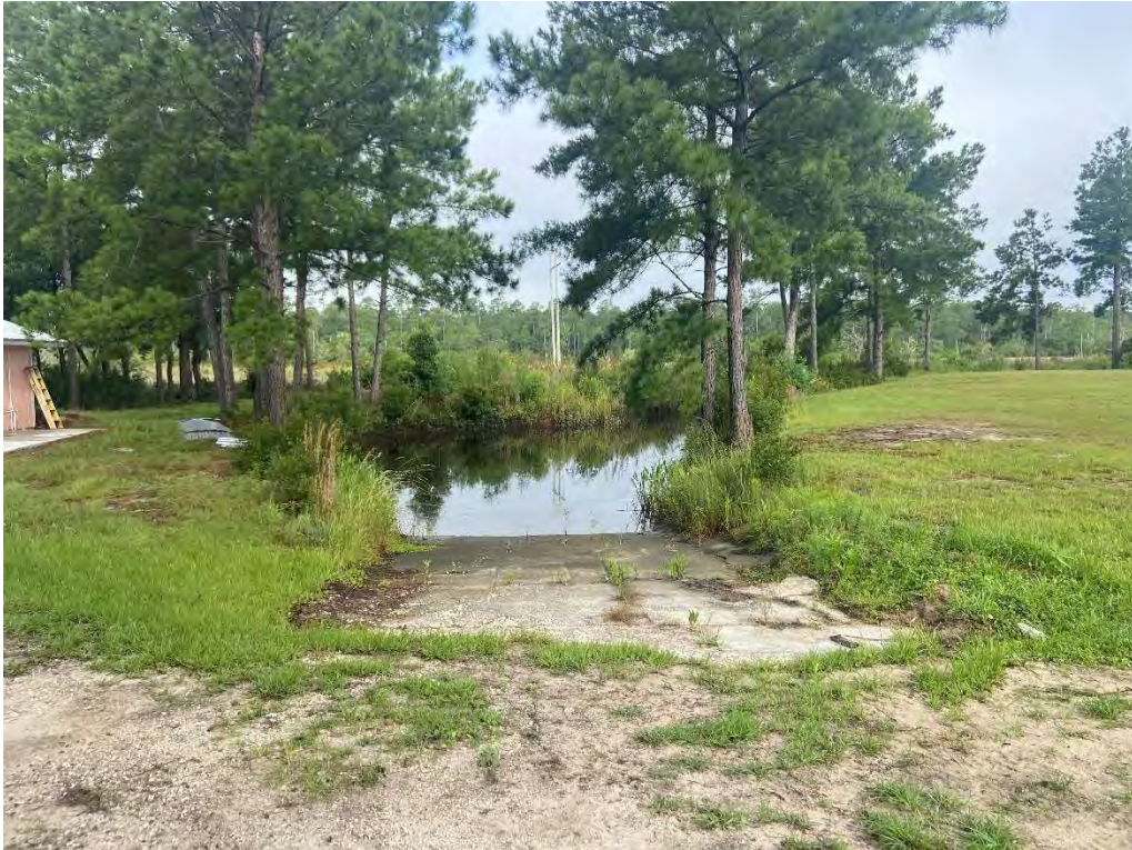
Photo 17: Facing west at concrete boat ramp located southwest of the basin
