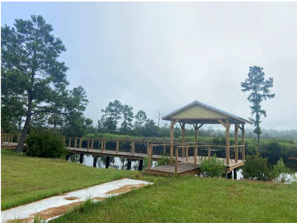
Photo 4: Facing north at pavilion, end of concrete pathway, and eastern access point
