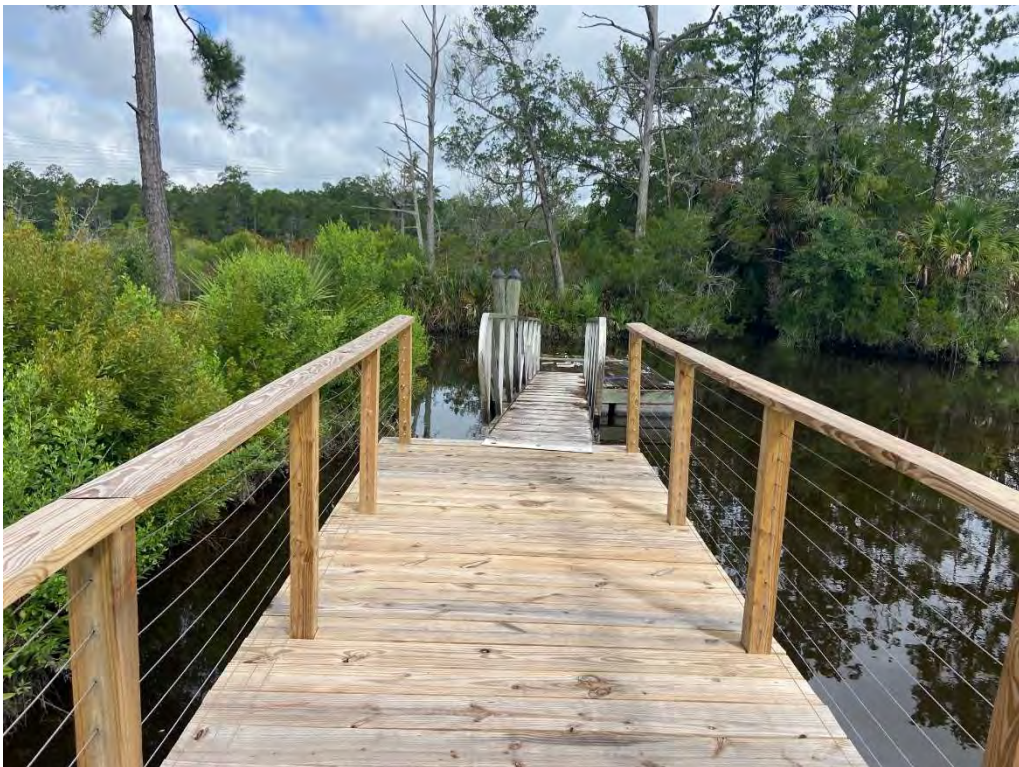
Photo 10: Facing west at end of wooden dock, aluminum ramp, and floating dock
