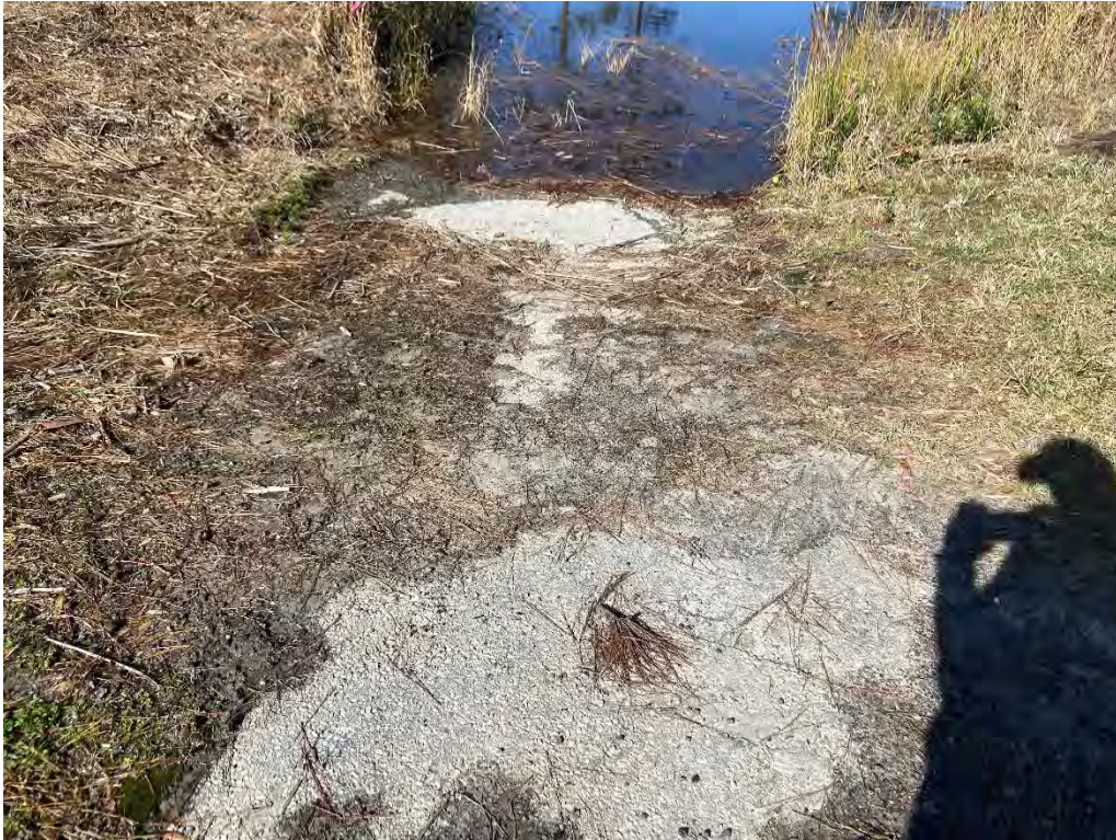
Photo 15: Facing north at asphalt boat ramp located in the southeast corner of the basin
