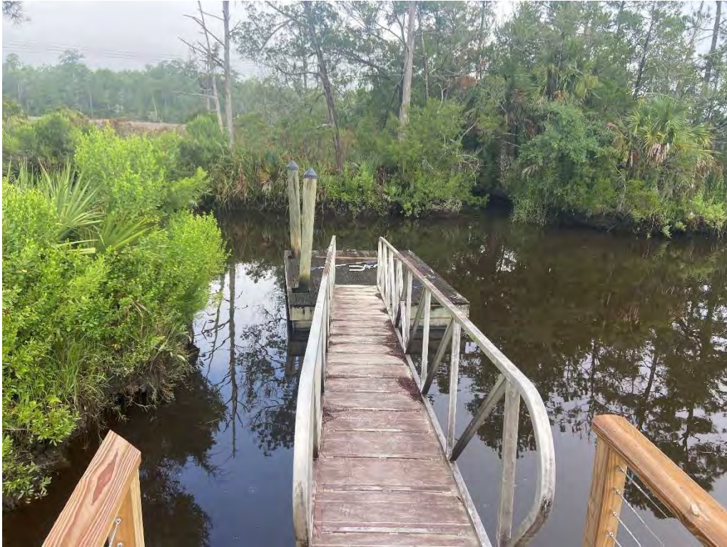
Photo 11: Facing west down aluminum ramp at floating dock
