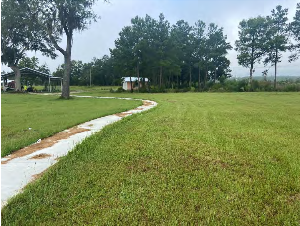
Photo 3: Facing south at concrete pathway away from dock
