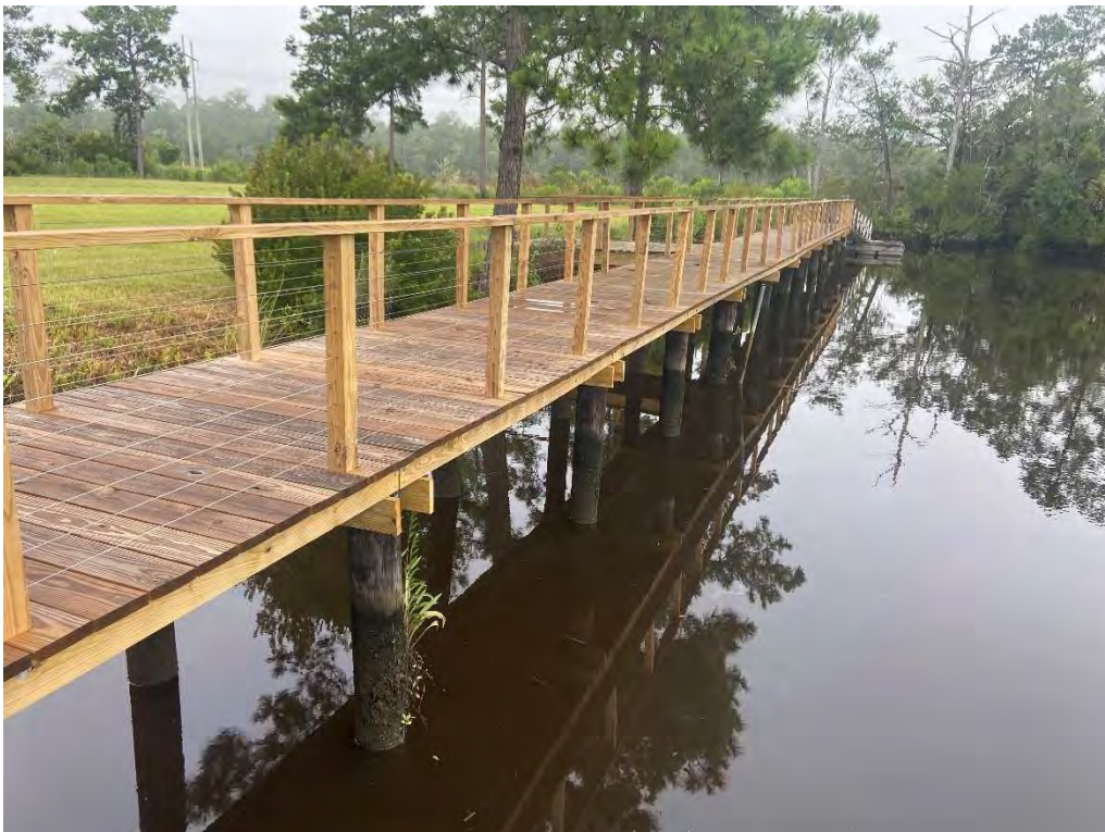
Photo 6: Facing west from pavilion at wooden dock
