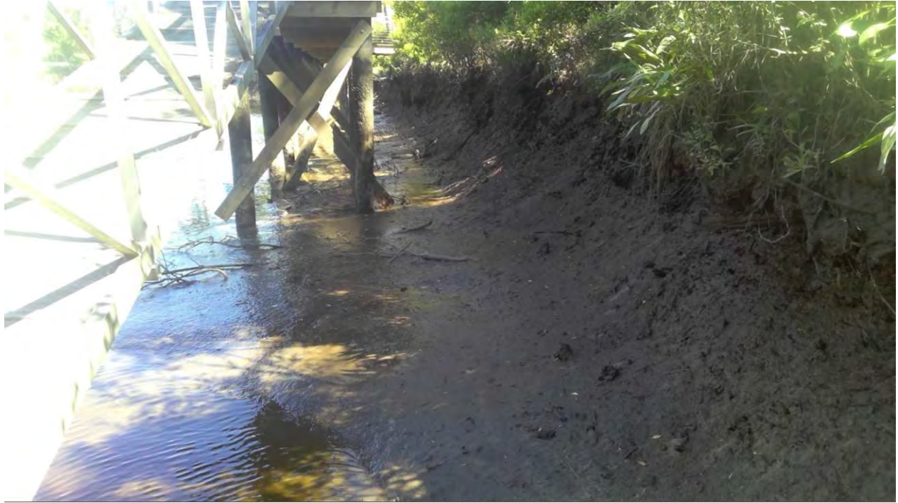
Photo 13: Facing east from floating dock at underside of wooden dock
