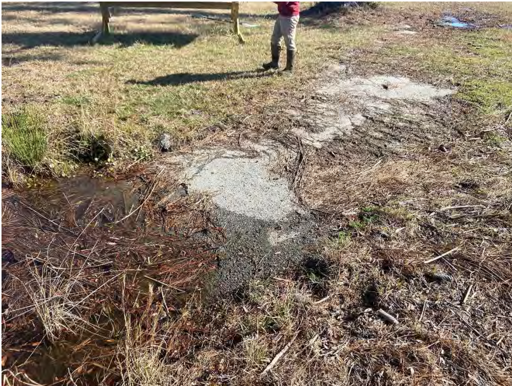
Photo 14: Facing east at asphalt boat ramp located in the southeast corner of the basin
