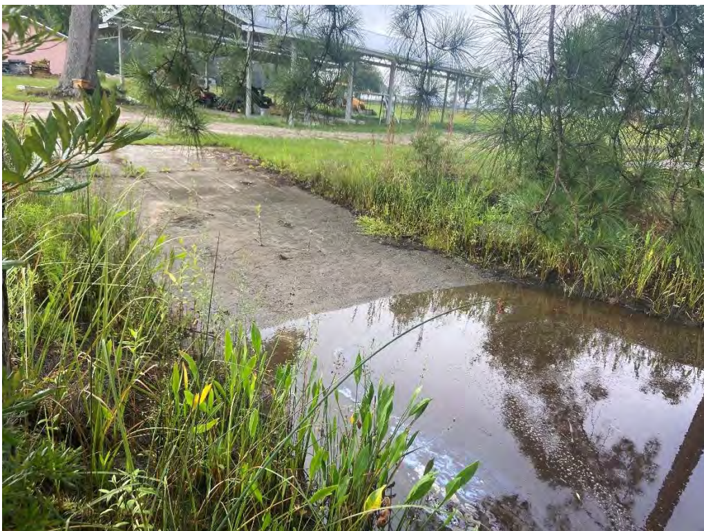
Photo 18: Facing south at concrete boat ramp located southwest of the basin
