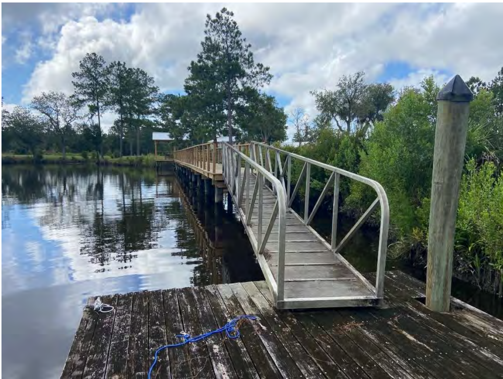
Photo 12: Facing east from floating dock at aluminum ramp and wooden dock
