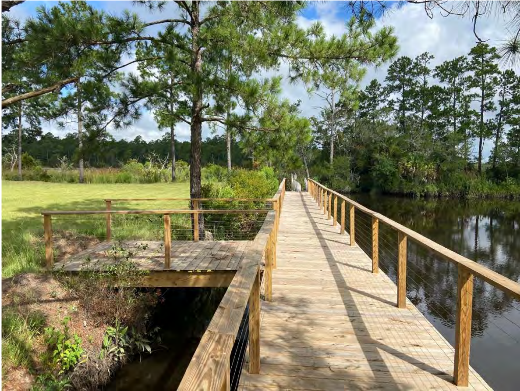
Photo 7: Facing west at wooden dock and western access point
