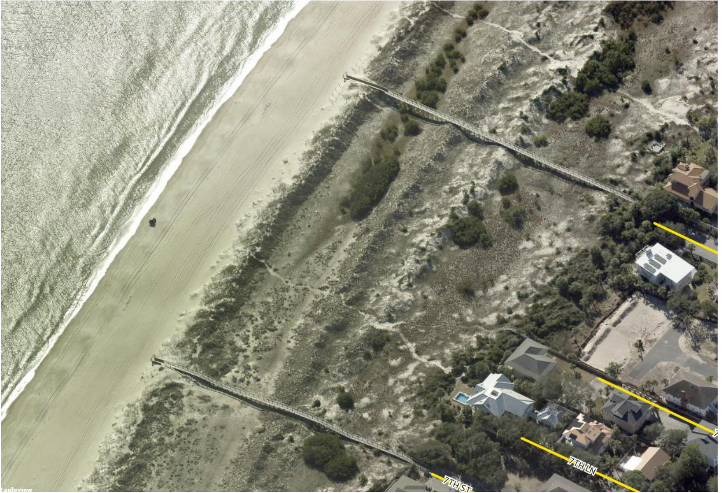
708 Butler Avenue, Atlantic Ocean, Tybee Island, Chatham Shared Dune Crosswalk
