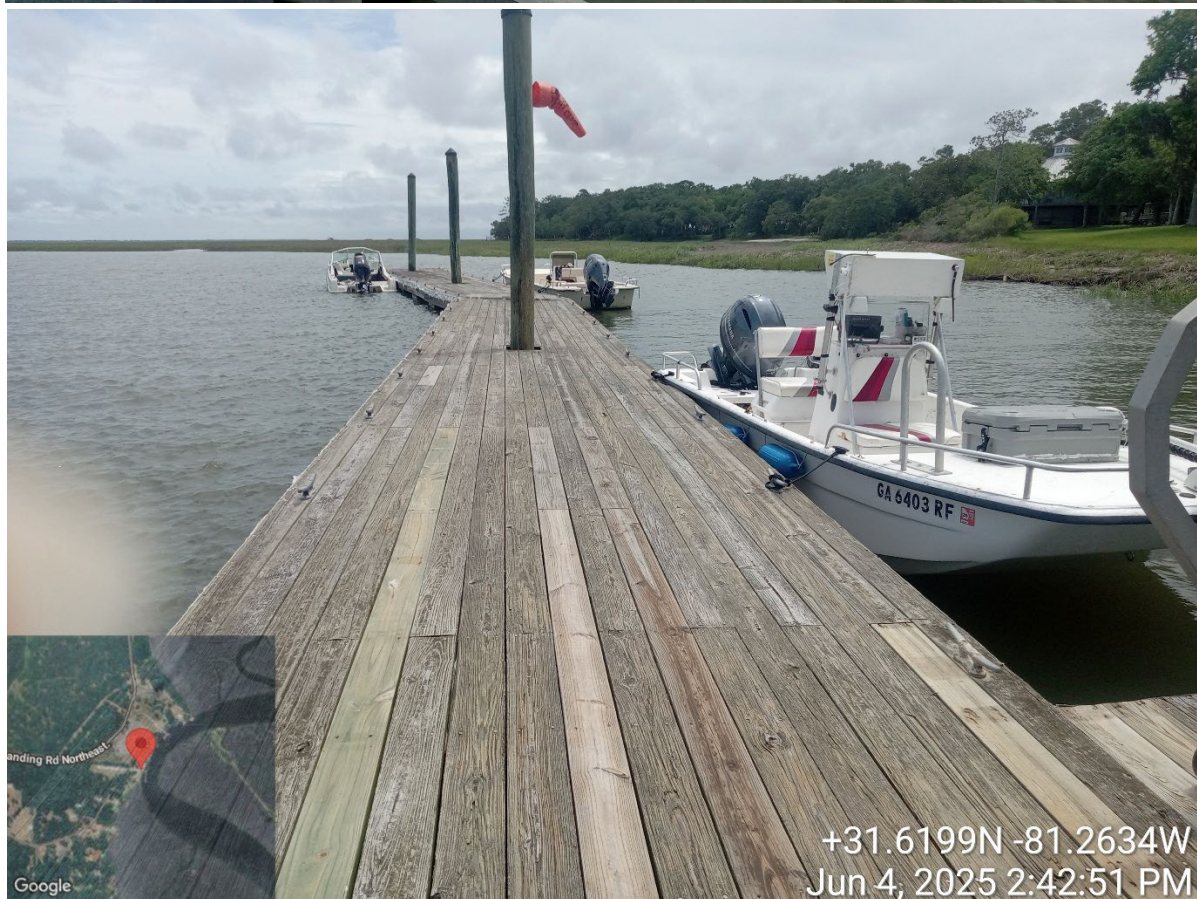
Site Visit – Barbour River Club Dock CMP20250018 – PM: Cheyenne Osborne and Mariana S.
