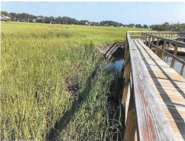
Photo 5: Erosion associated with channel migration
