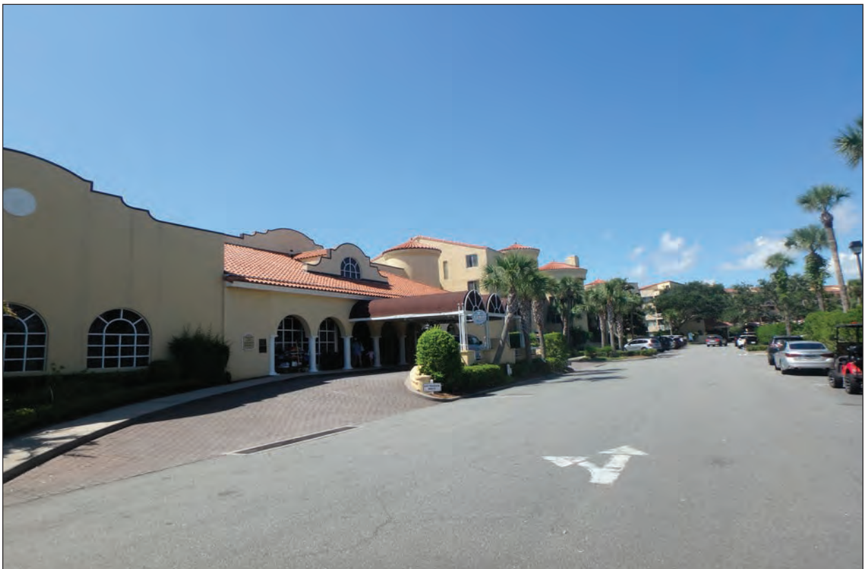
Figure 4.11 Southeastern view of The King and Prince Hotel (NRHP #04001465), northwest elevation, central atrium.
