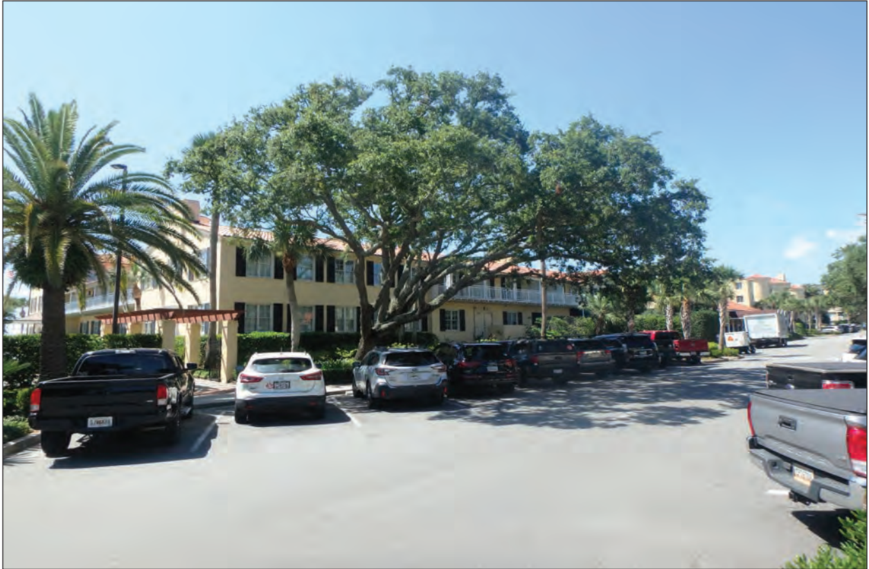
Figure 4.12 South oblique view of The King and Prince Hotel (NRHP #04001465), northwestern corner.
