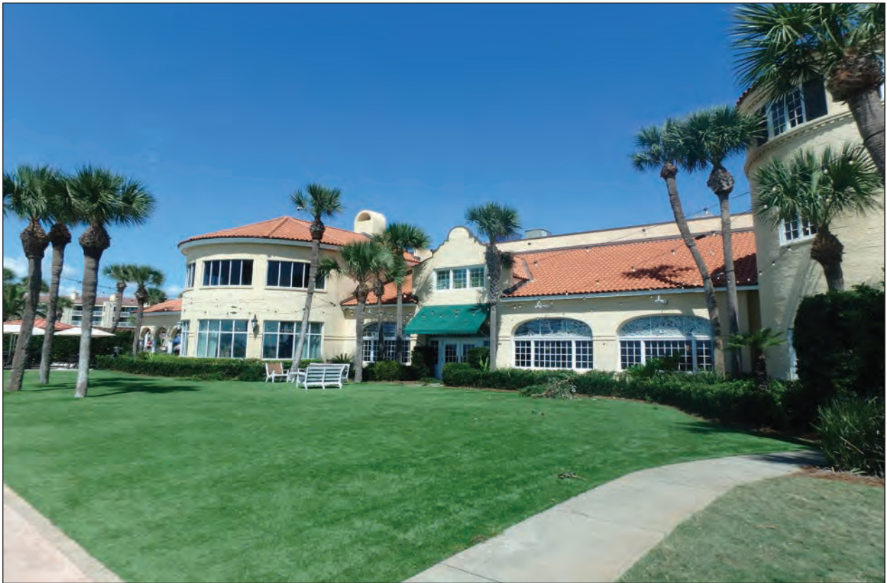
Figure 4.14 Western view of The King and Prince Hotel (NRHP #04001465), southeast elevation, central atrium.
