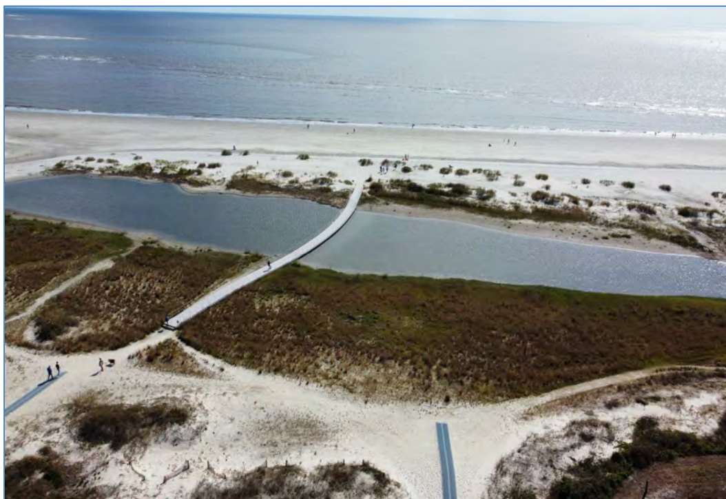
Wetland 3 and Tidal Pool 1 southern pool area – facing east
