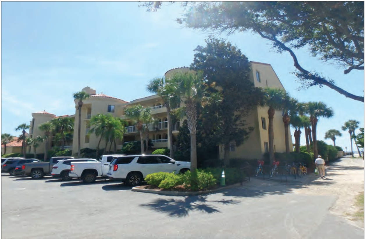
Figure 4.10 Eastern view of The King and Prince Hotel (NRHP #04001465), northwest elevation, southwestern corner.
