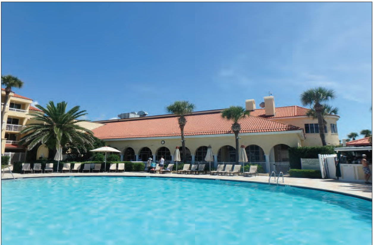
Figure 4.15 Northeastern view of The King and Prince Hotel (NRHP #04001465), central atrium.
