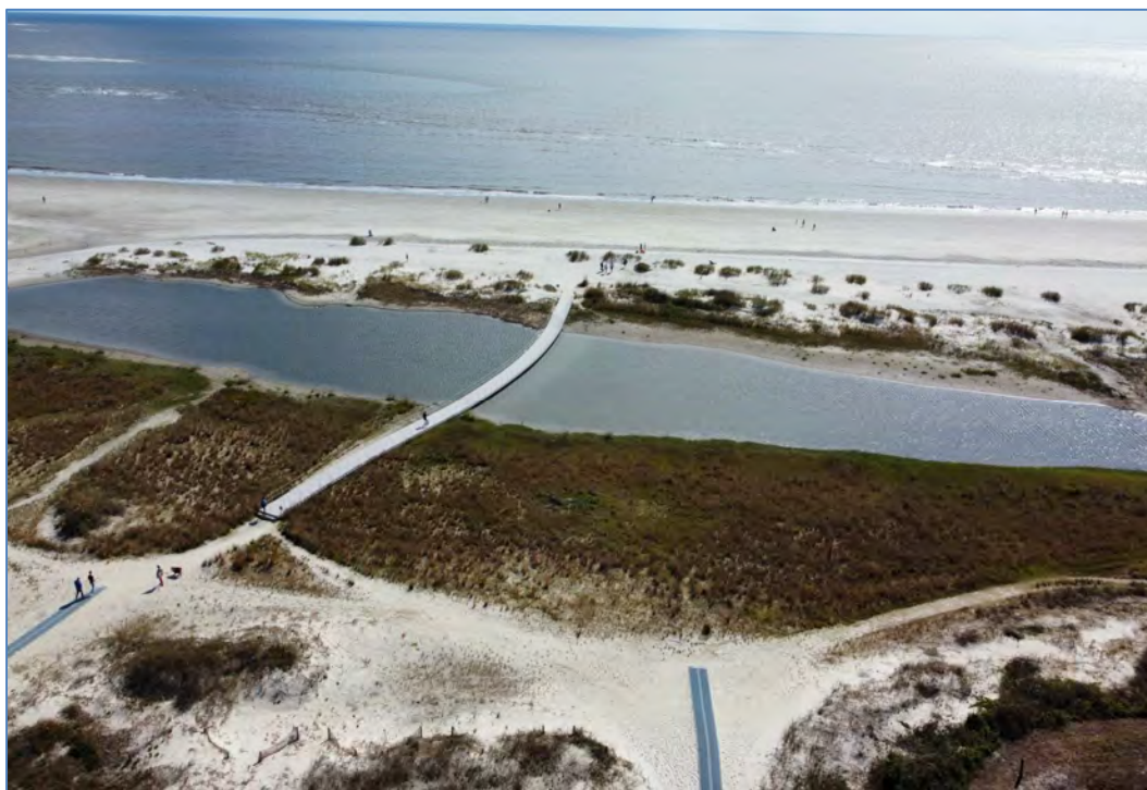
Wetland 3 and Tidal Pool 1 southern pool area – facing east
