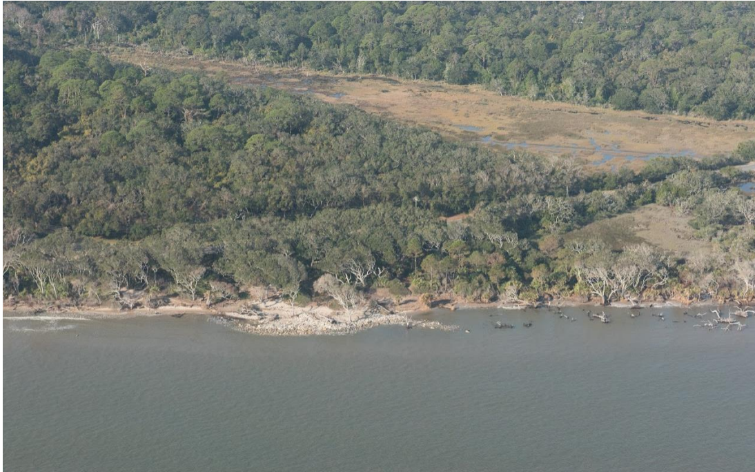
Exhibit 3. Eroded conditions north of existing revetment limits at Driftwood Beach during King tide conditions
