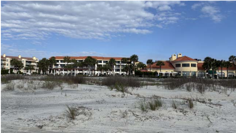
3 VIEW OF THE SEAWARD-MOST DUNE ALONG THE BEACH FRONT OF THE HOTEL
