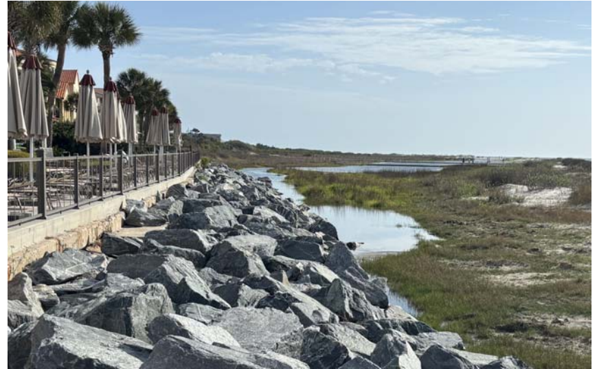
2 VIEW OF WATER IMPOUND AREA ALONG THE BEACH FRONT OF THE HOTEL
