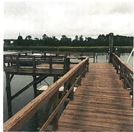
Photo 5: Existing walkway and deck
