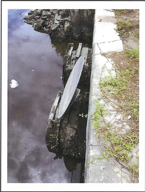
West Culvert: South side looking west
