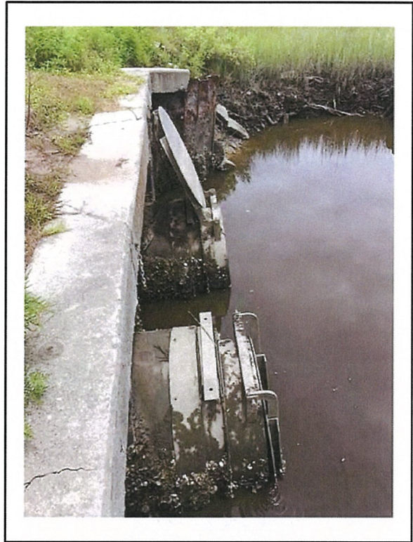
West Culvert: South side looking east
