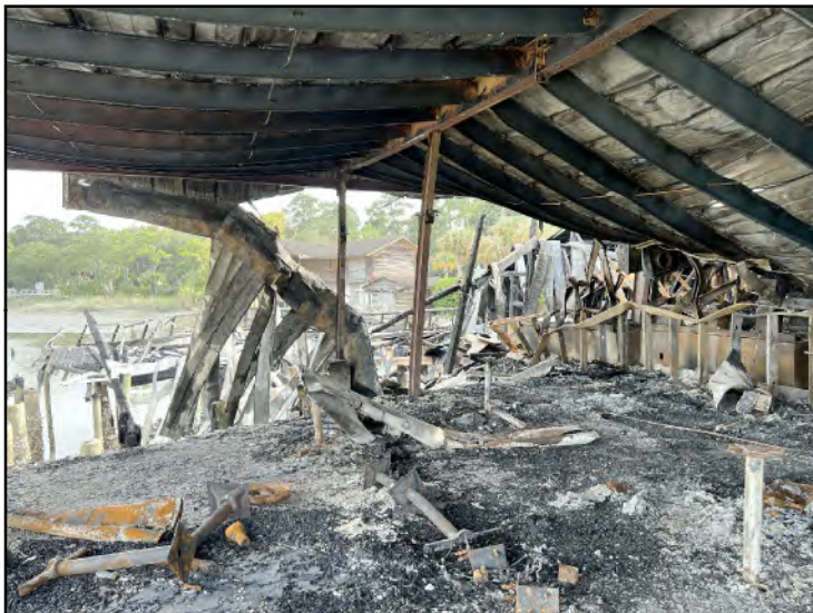
Photo 3: Existing restaurant condition
