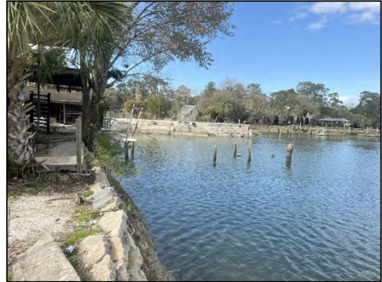
Photo 2: Existing wall behind building on Project Area A
