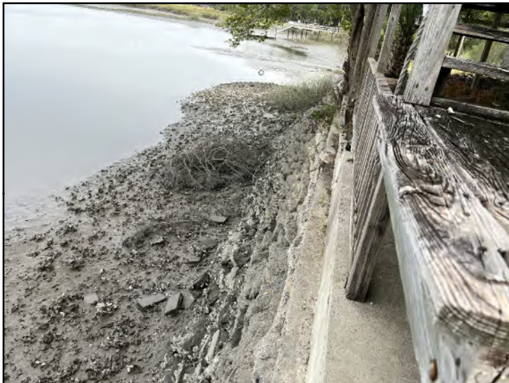
Photo 7: Existing bulkhead at 7012 LaRoche Avenue
