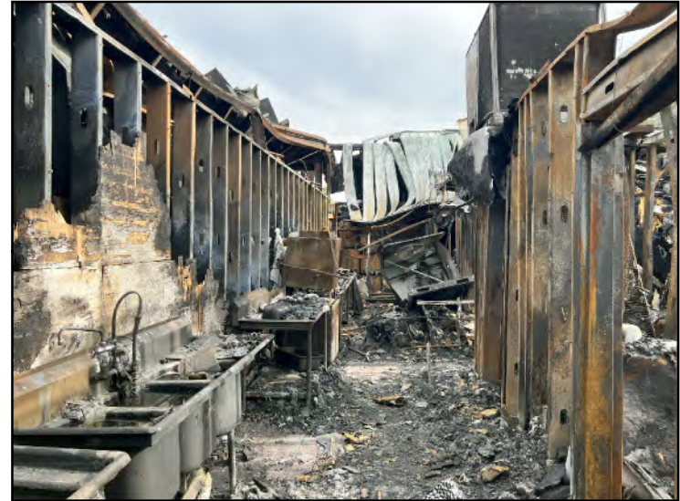
Photo 2: Existing restaurant condition
