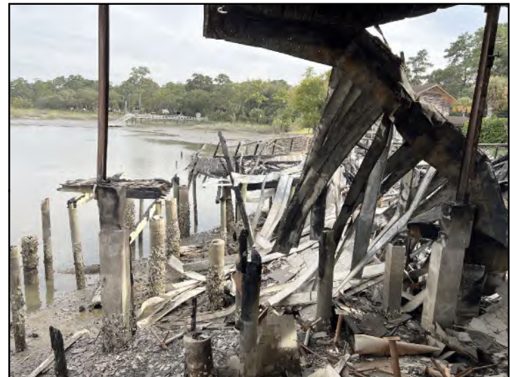
Photo 4: Existing restaurant condition
