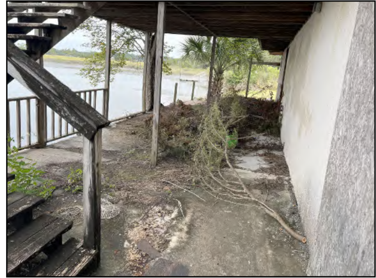
Photo 6: Adjacent building at 7012 LaRoche Avenue to be demolished
