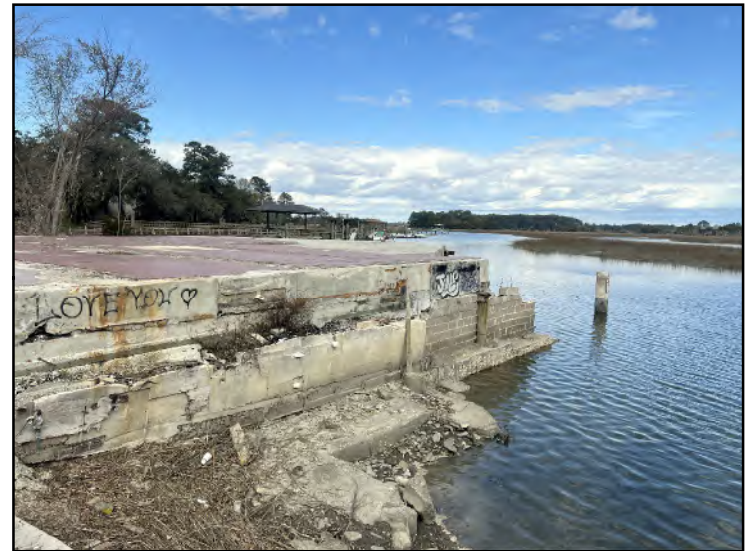
Photo 4: Concrete slab and wall within Project Area A
