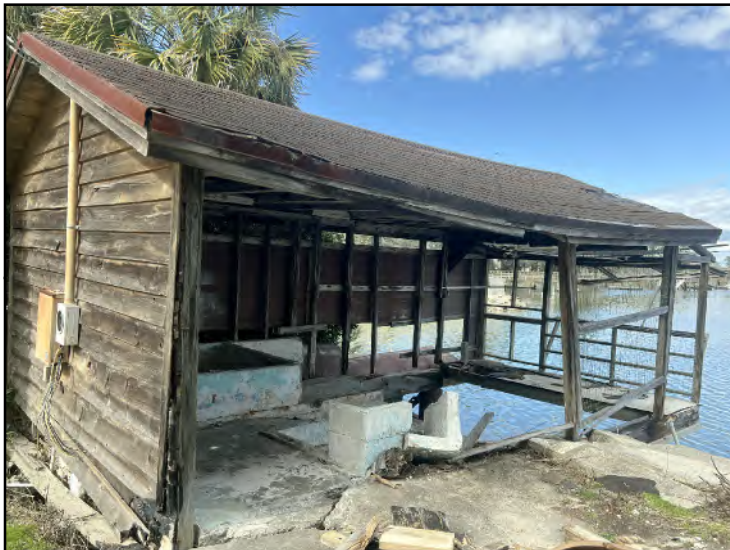
Photo 3: Existing structure over water
