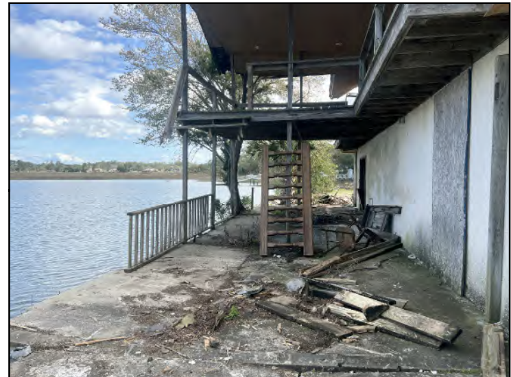
Photo 4: Rear of existing building
