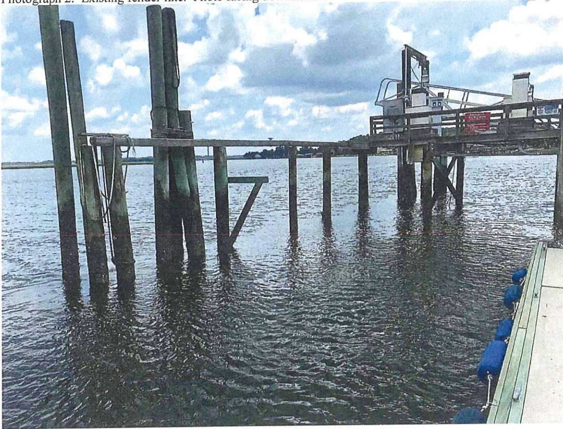
Photograph 2: Existing fender line. Photo facing downstream
