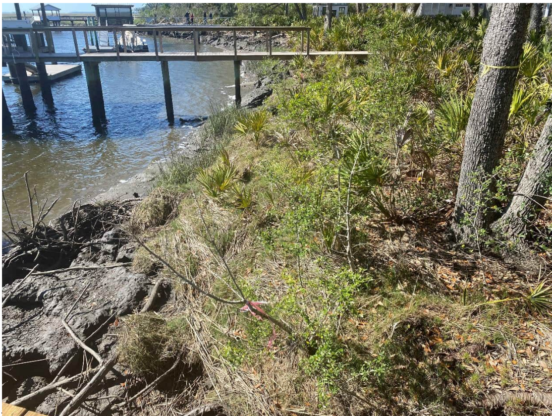
Photo 2: DNR and CE line within Lot 1, facing south
