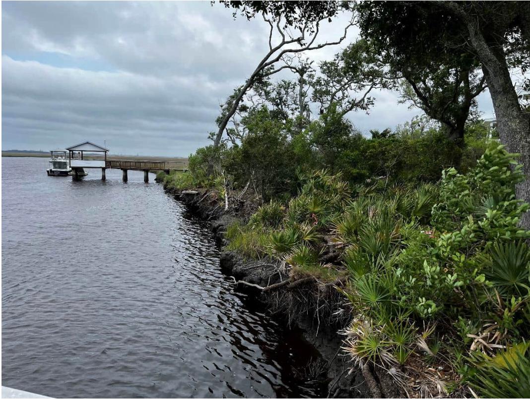
Photo 1: DNR and CE line within Lot 4, facing south
