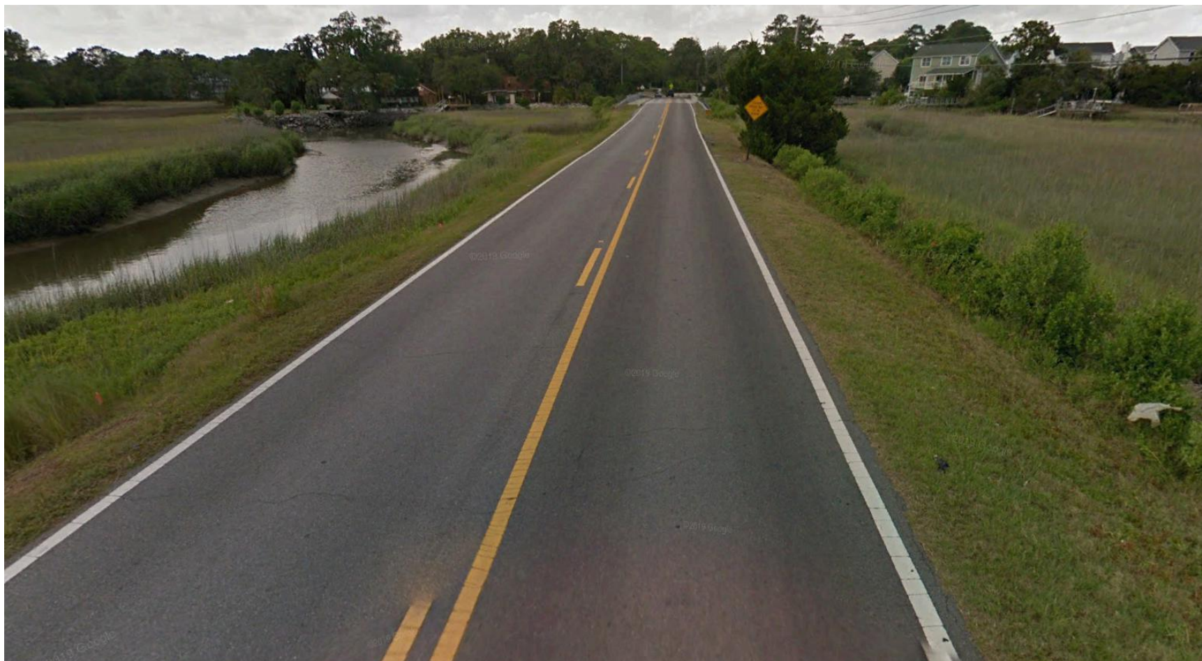
Looking north towards bridge with Betz Creek adjacent to southbound travel lane
