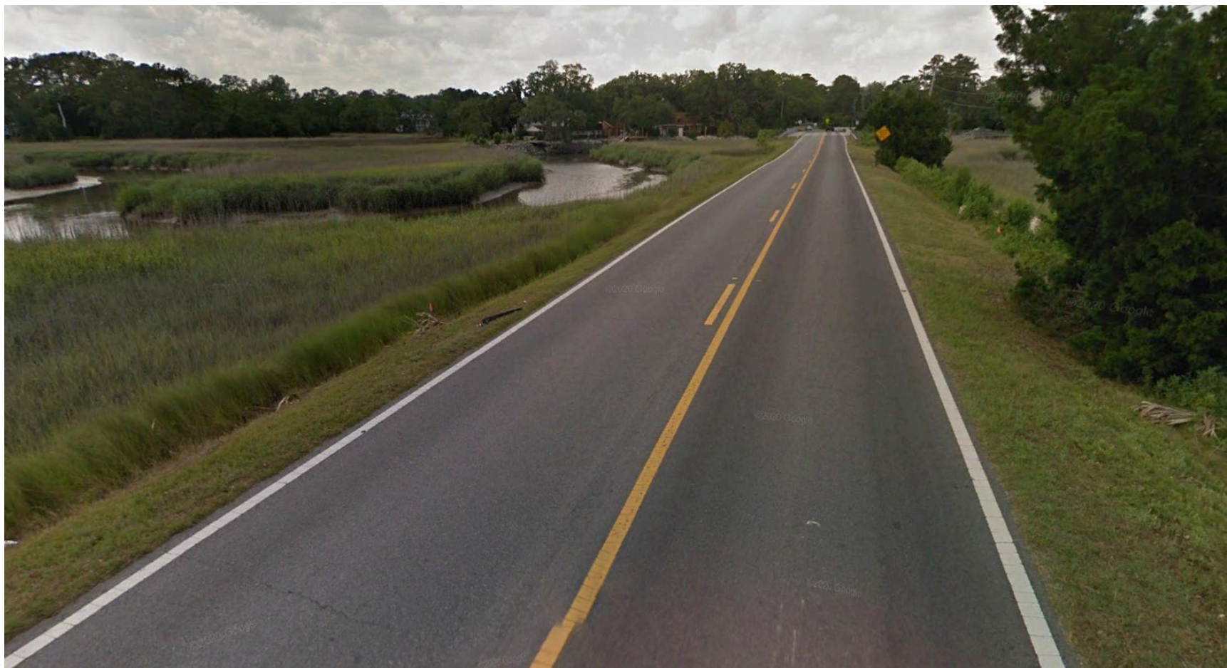
Looking north towards Walthour Road Bridge over Betz Creek
