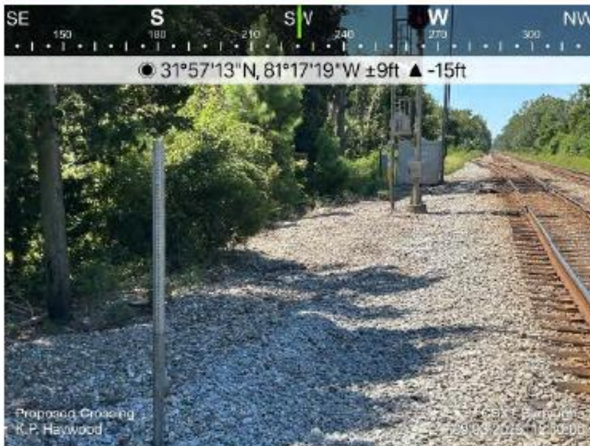
Guide Piles to be Removed K.P. Haywood
