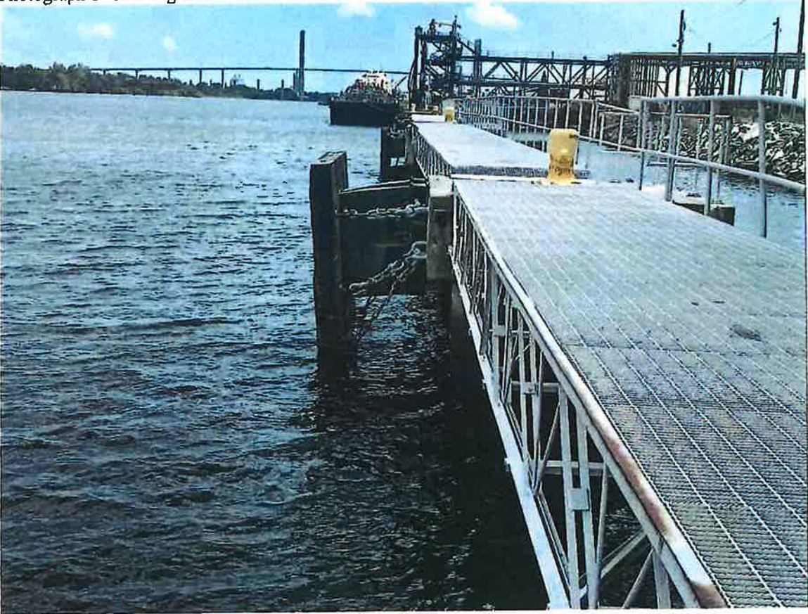
Photograph 1: Existing fenders and bollards on downstream end of the dock
