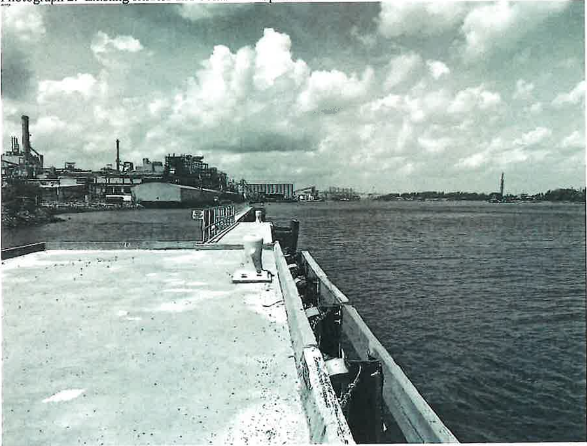
Photograph 2: Existing fenders and bollards on upstream end of the dock
