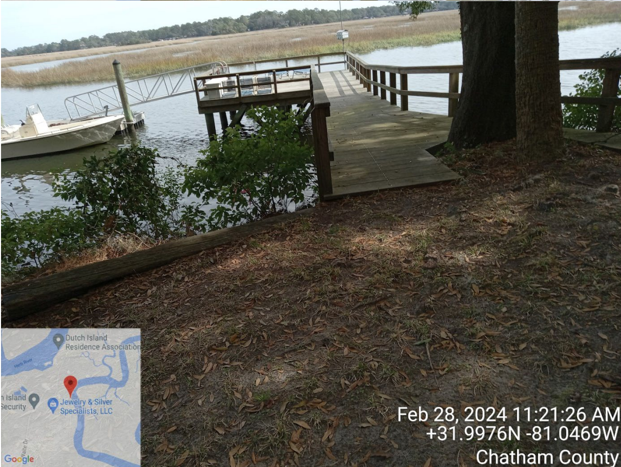
110 Herb River Dr. – Henry Smith Lewis – Install Timber Bulkhead by Cheyenne Osborne
