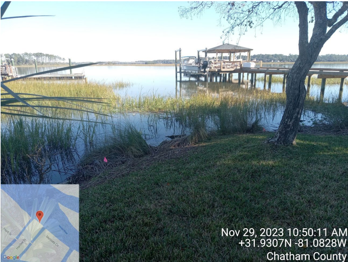
Site Visit – 11.29.23 – 13 Hardee Drive – Chuck Hartman – CMPA Bulkhead along Moon River By Cheyenne Osborne w/ Maitland Bass
