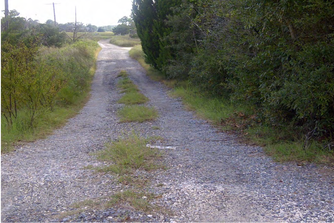
Photograph 1: This picture was taken from the intersection of Highway 80 and Polk Street. Note elevation change in rear of picture.
