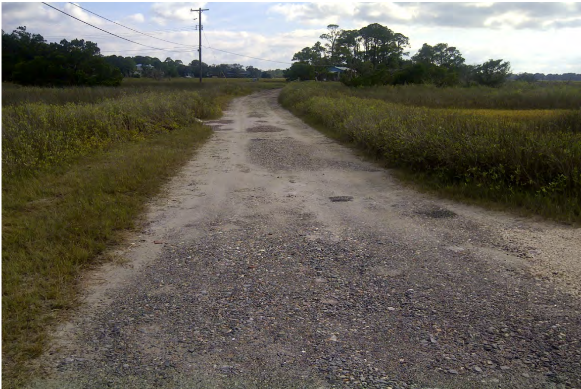
Photograph 2: Typical condition of project area where raising of existing roadway will occur.
