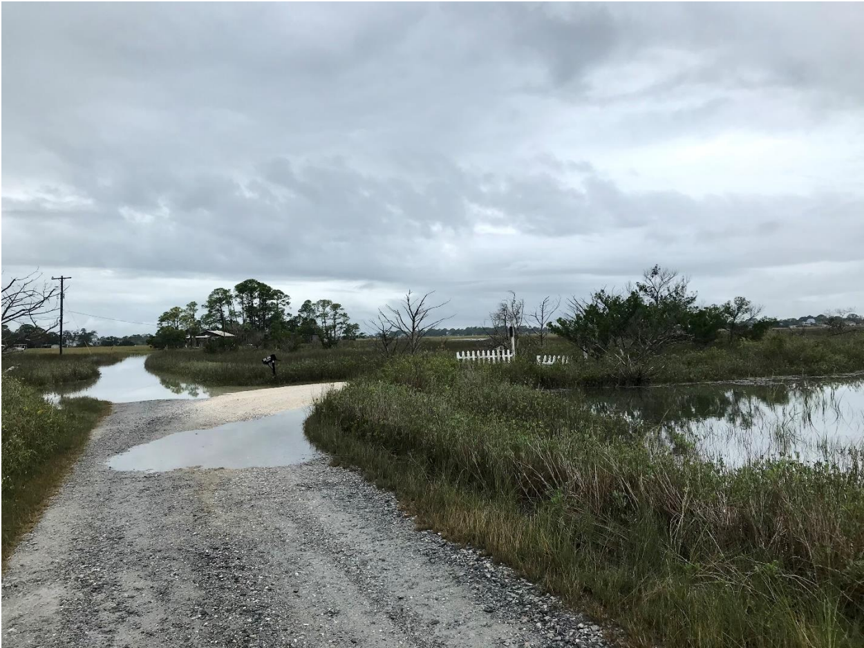
October 21, 2020 around High Tide: Looking south from Polk Street ROW toward Leonard Residence
