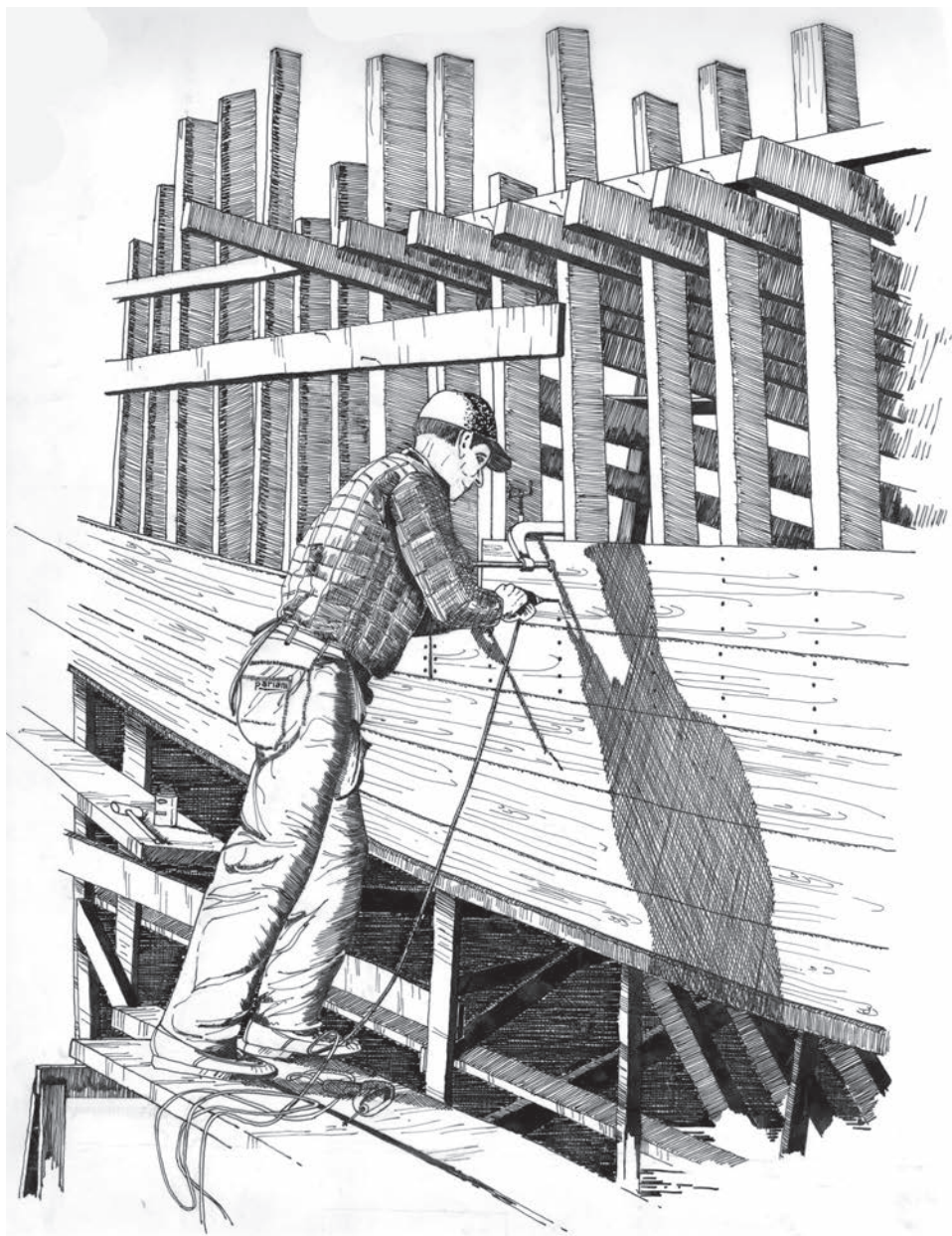
An illustration of a shrimp trawler being constructed, reprinted from "Coastlines Georgia," Vol. 3, No. 4, July-August 1980. Artwork by Rick Pariani.
