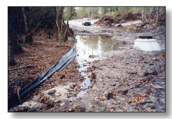
Figure 2.2.2.2a Failed Sediment Control Fence
